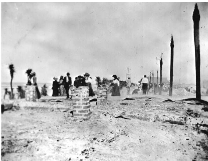
Clarendon Hotel site after fire.
