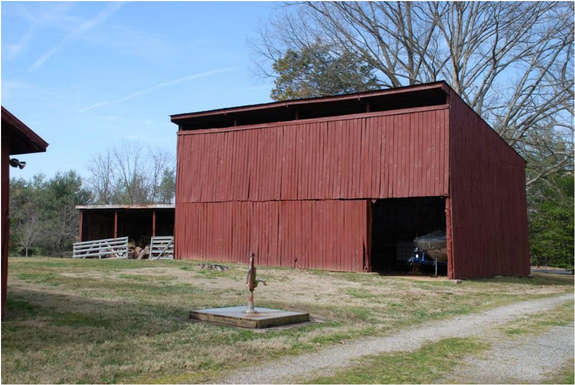
Photo 27: Pole Barn #1, Bel Air, 03/07/2012
