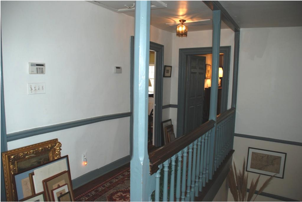
Photo 13: Second floor landing, Bel Air, 03/07/2012
