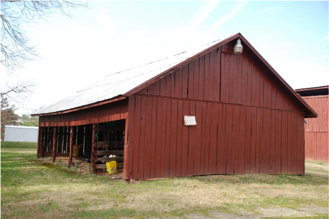
Photo 28: Pole Barn #2, Bel Air, 03/07/2012
