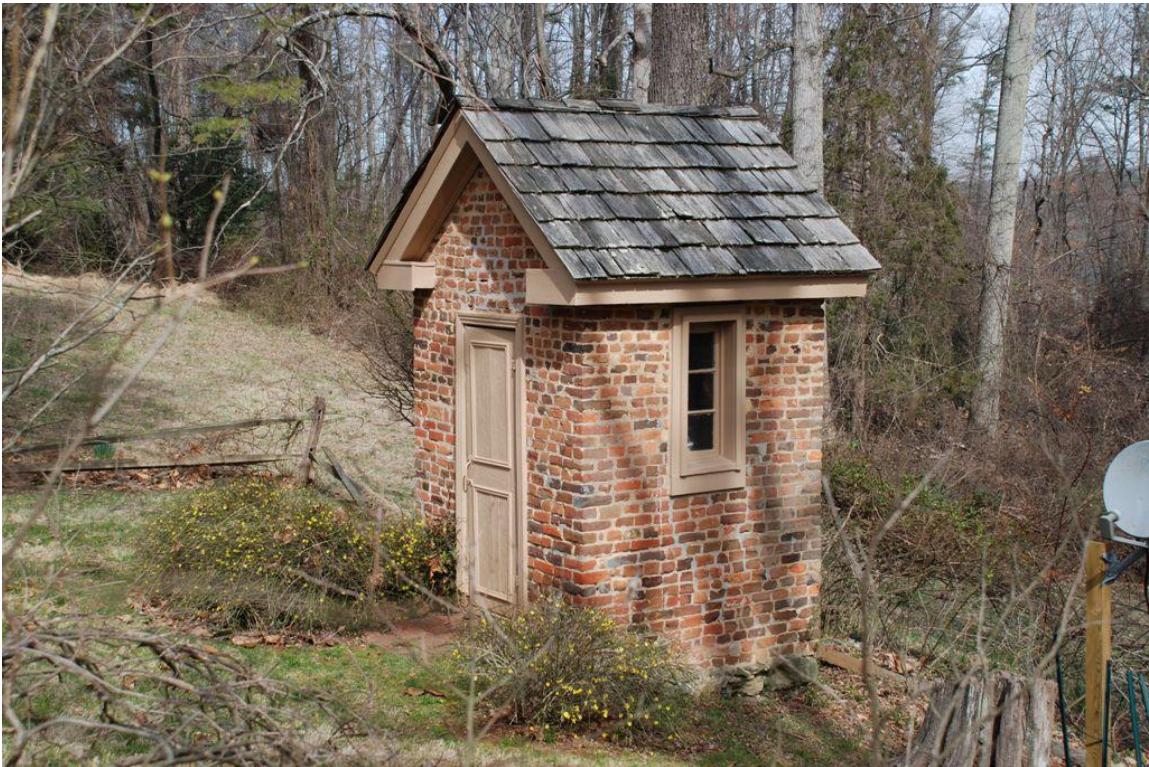
Photo 24: Brick storage building/ privy, Bel Air, 03/07/2012
