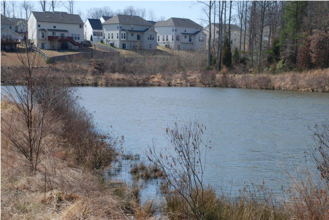
Photo 34: Adjacent neighborhood retention pond (partially on easement property), Bel Air, 03/07/2012
