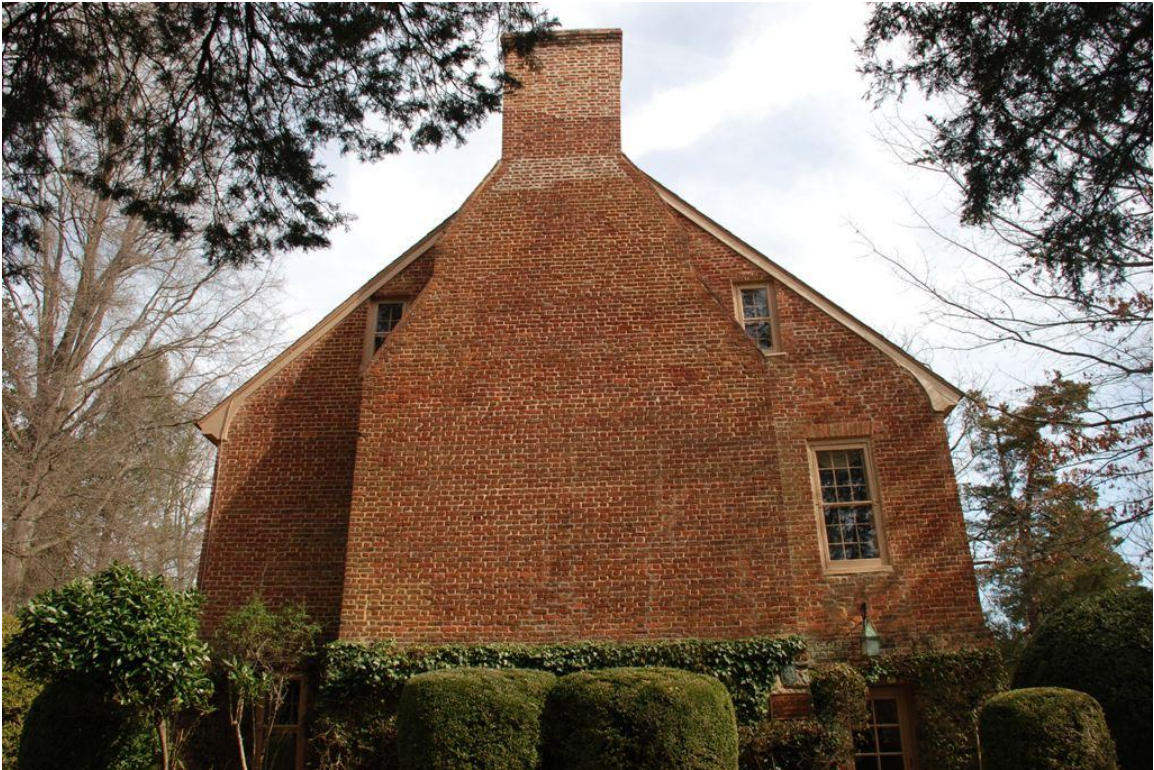
Photo 4: South elevation, Main House, Bel Air, 03/07/2012
