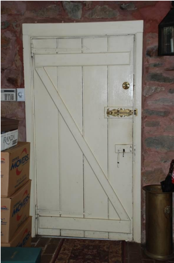
Photo 21: Exterior basement door, Bel Air, 03/07/2012
