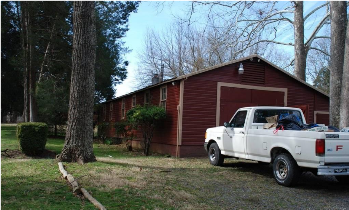
Photo 25: Garage/ storage/ office building, north elevation, Bel Air, 03/07/2012
