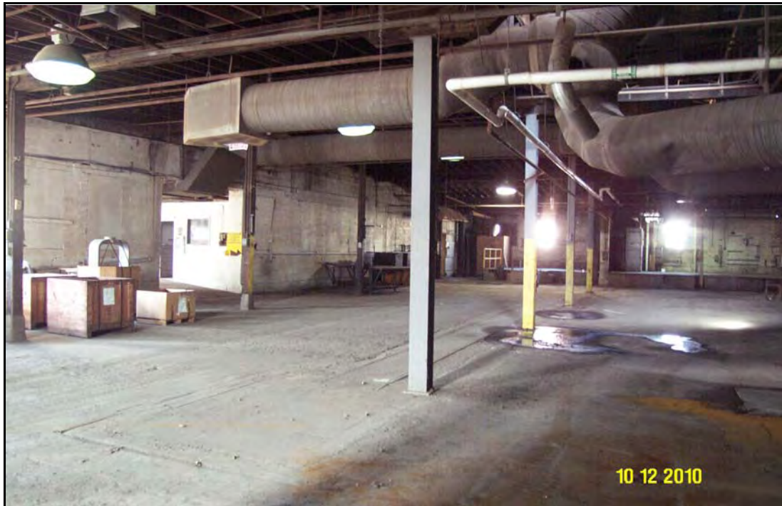
An interior view of the foundry.
