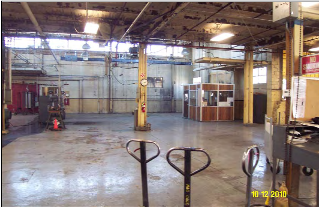
A view of another middle section of the plant.
