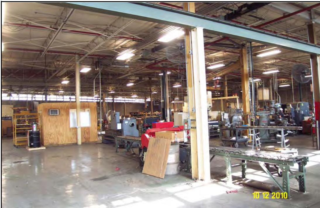
A view of the westerly concrete block addition to the plant.
