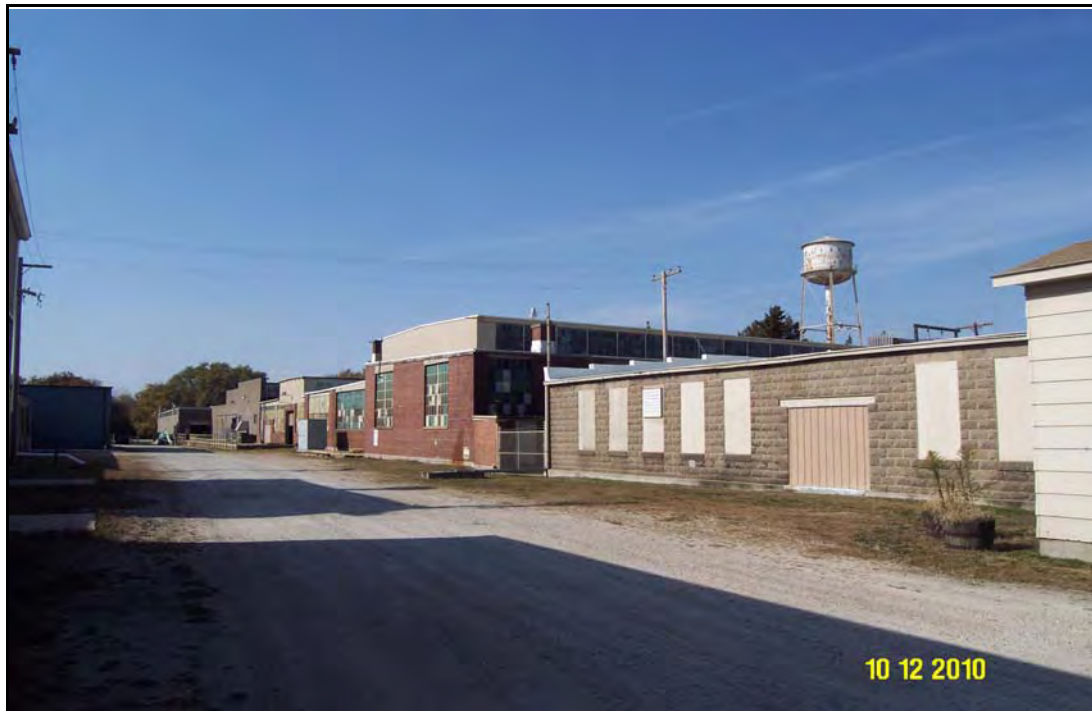
A view of the main plant looking northwesterly.
