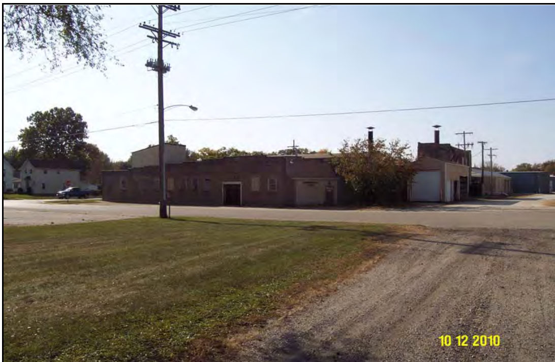
A front view of the foundry looking southwesterly.
