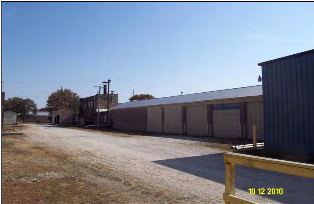
A rear view of the foundry and sand storage bays looking southeasterly.
