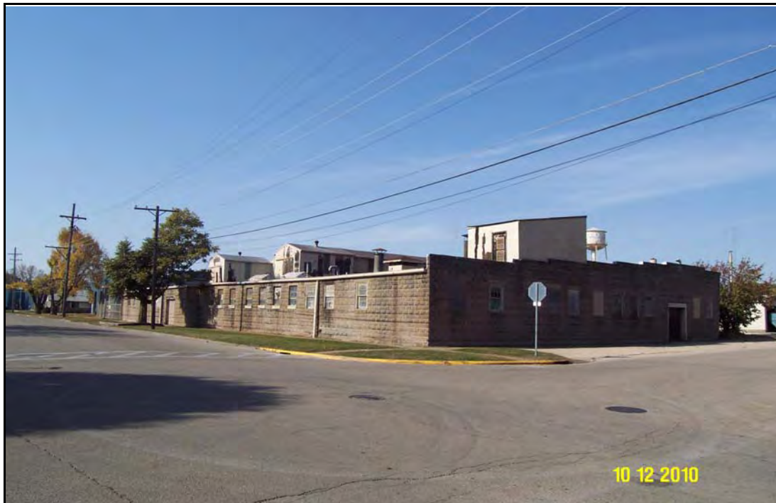
A rear view of the foundry looking northwesterly.
