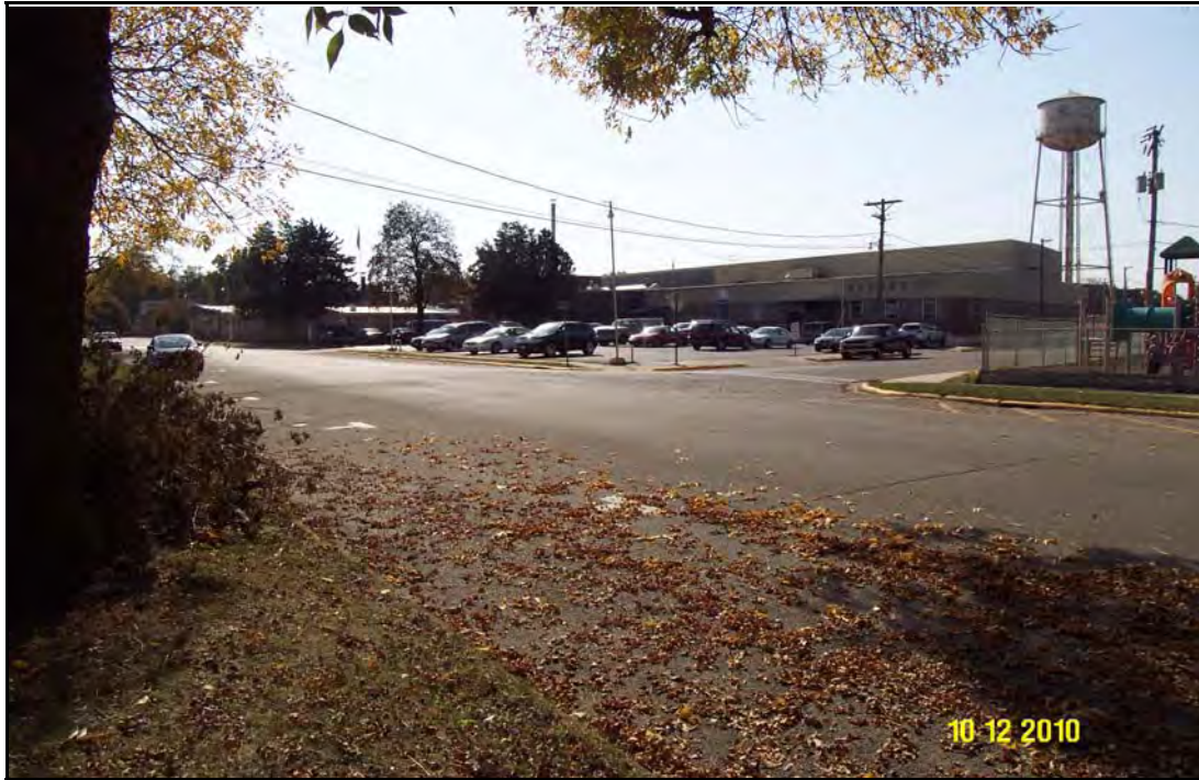
A view of the main plant looking westerly.
