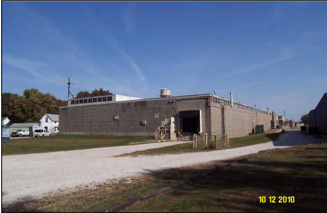
A rear view of the main plant looking easterly.
