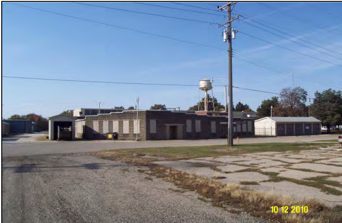
A view of the maintenance addition and storage buildings looking westerly.
