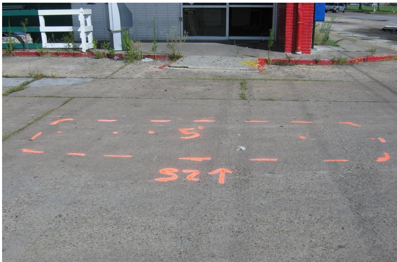
#2- This is the area of the scan #2 in front of the main doors.
