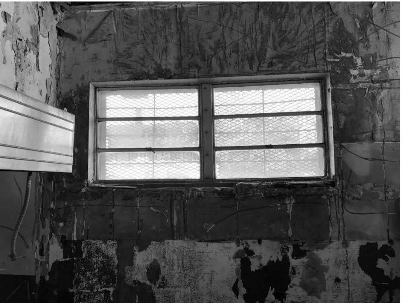
15. REPAIR & RESTORE EXISTING WINDOW FRAMES & INT. FINISHED HEAD/JAMBS/SILL. REPLACE COMPONENTS TO MATCH WHERE REQ'D.
