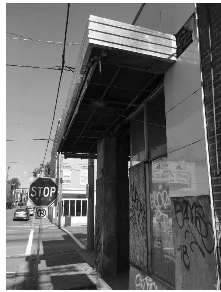
9. SALVAGE EXISTING TILE CLADDING AND (1) PROVIDE REPLICA MATERIAL TO MATCH OR (2) PROVIDE ALL NEW SIMILAR CLADDING MATERIAL
