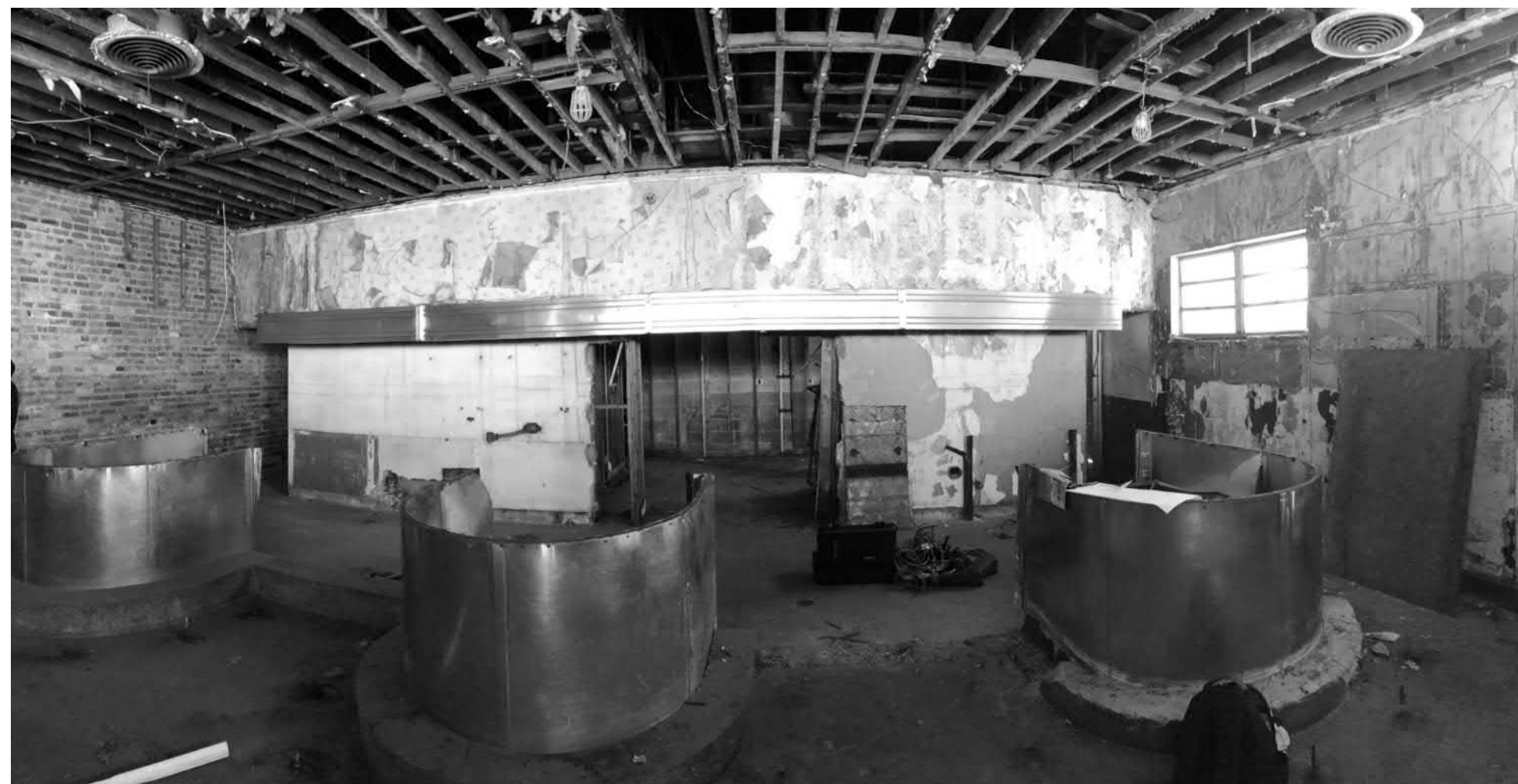
17. REPAIR & RESTORE INTERIOR FINISHES & PREP TO RECEIVE NEW CONSTRUCTION.
