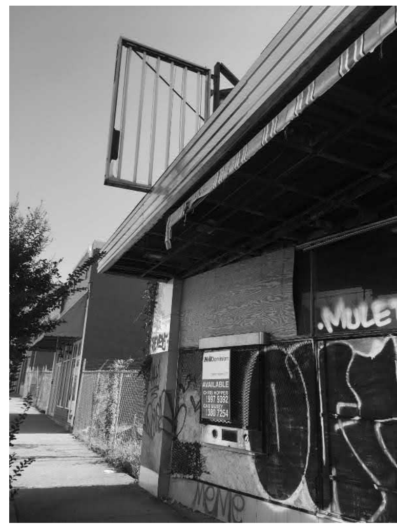
7. REMOVE EXISTING TRANSACTION WINDOW & SHEATHING. REPAIR & PREP STOREFRONT FOR NEW COMPONENTS.
