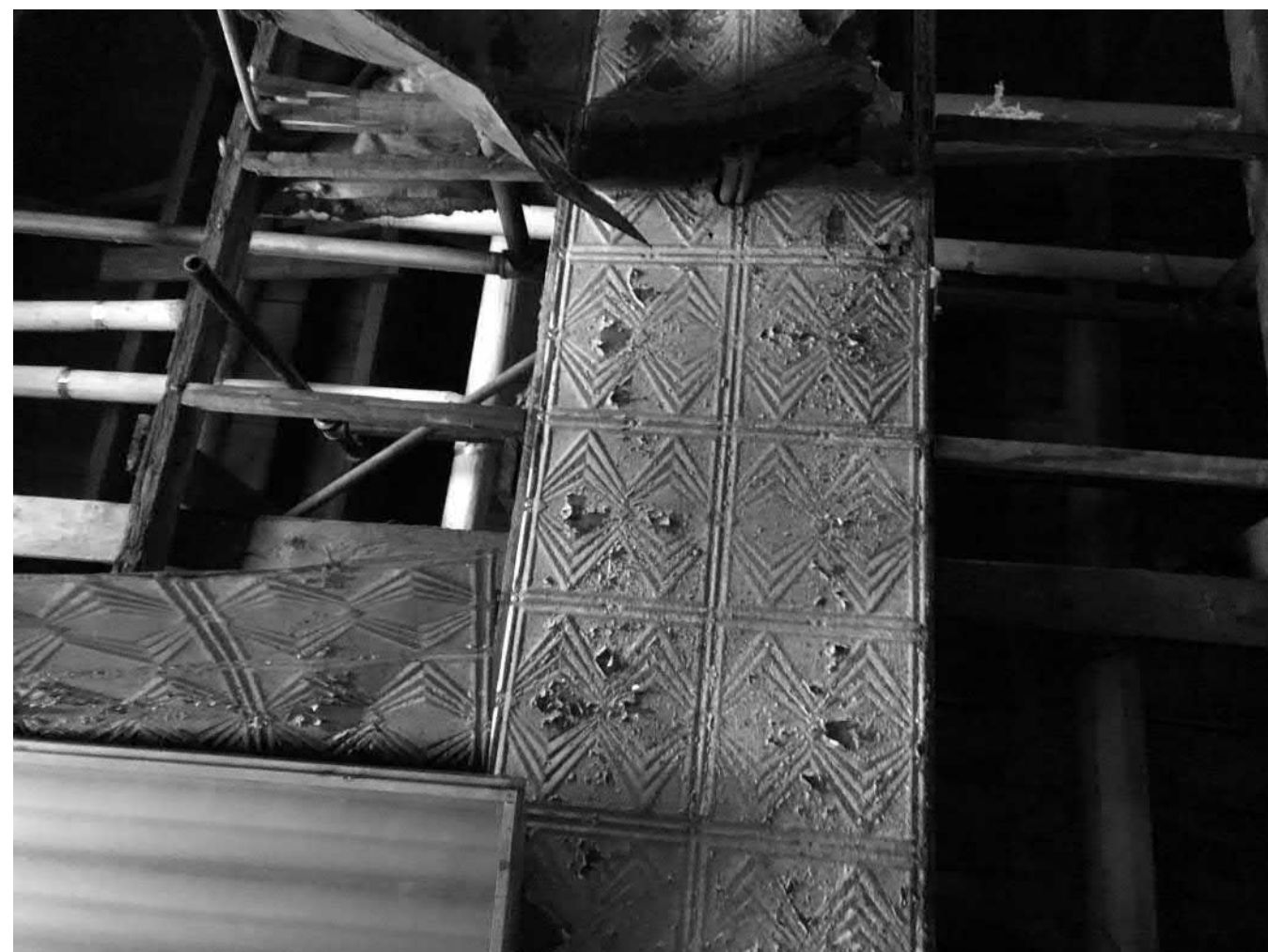
16. SALVAGE, REPAIR, & RESTORE STAMPED MTL CEILING TILES. PROVIDE REPLICA TILES AS REQ'D.
