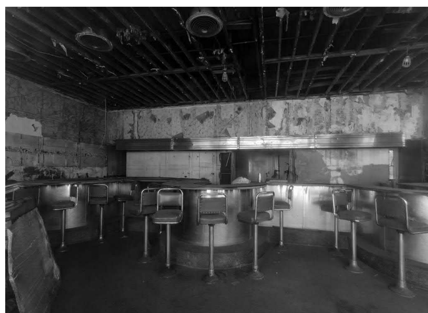
20. FOR REFERENCE: HISTORIC PHOTO OF SERVICE COUNTER.
