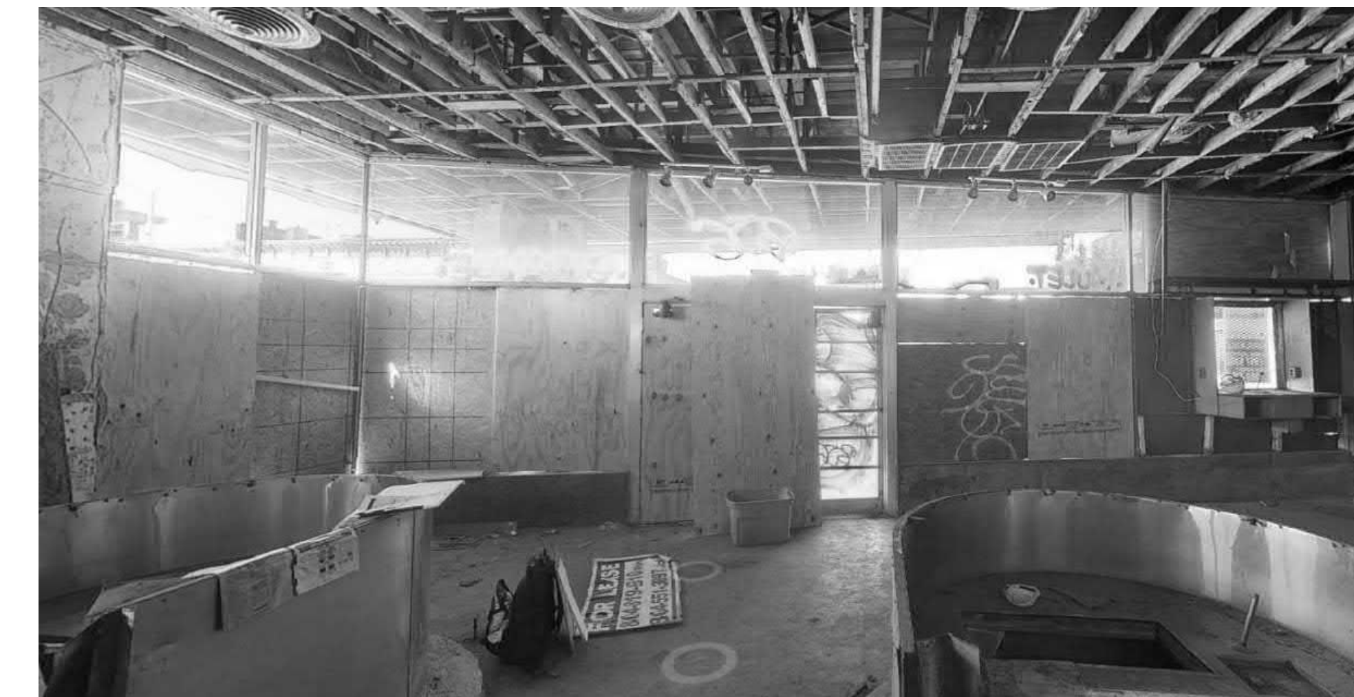
18. REPAIR & RESTORE STOREFRONT & INTERIOR SILL.
