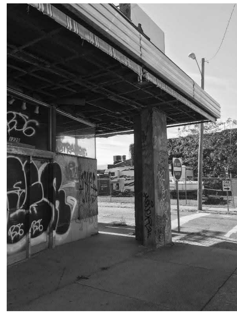
6. REMOVE EXISTING CANOPY SHADE, REPAIR, REPOINT, & RESHORE MASONRY COLUMN.
