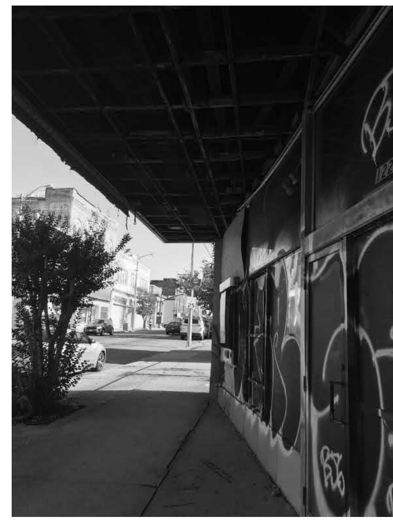
5. REPAIR & PREP CANOPY FRAMING TO RECEIVE NEW MATERIAL.
