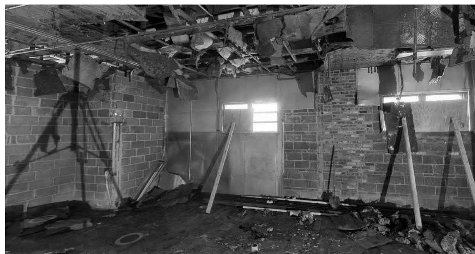
25. REPAIR INTERIOR FINISHES & PREP TO RECEIVE NEW CONSTRUCTION.
