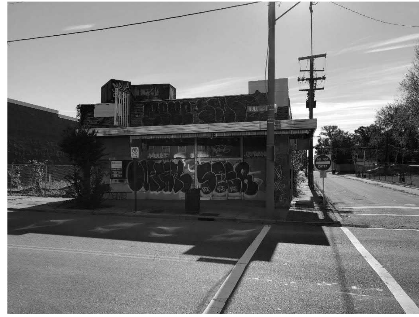
4. REPAIR & RESTORE EXISTING STOREFRONT & MTL CANOPY
