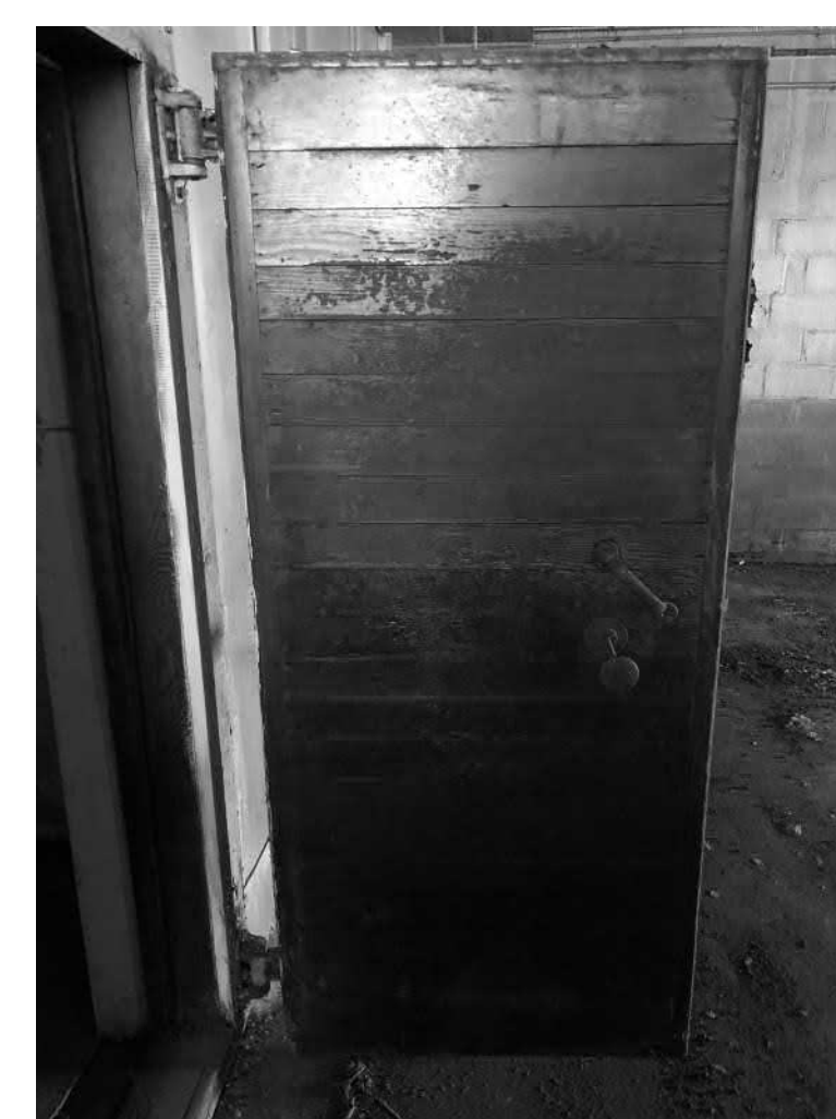
27. SALVAGE, REPAIR, & RESTORE LOCKER DOORS.
