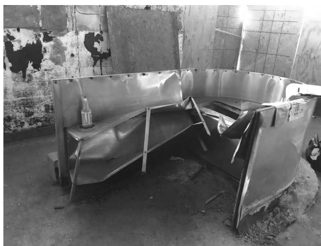
21. REPAIR DAMAGED COMPONENTS OF BOOTHS & COUNTERS. PROVIDE NEW, SIMILAR COMPONENTS WHERE REQ'D.
