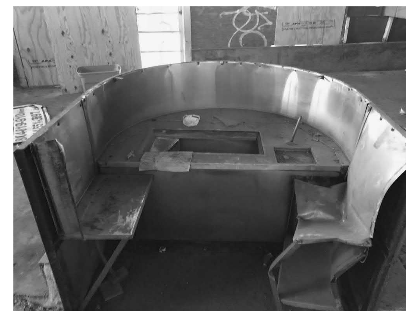
22. REPAIR DAMAGED COMPONENTS OF BOOTHS & COUNTERS. PROVIDE NEW, SIMILAR COMPONENTS WHERE REQ'D.
