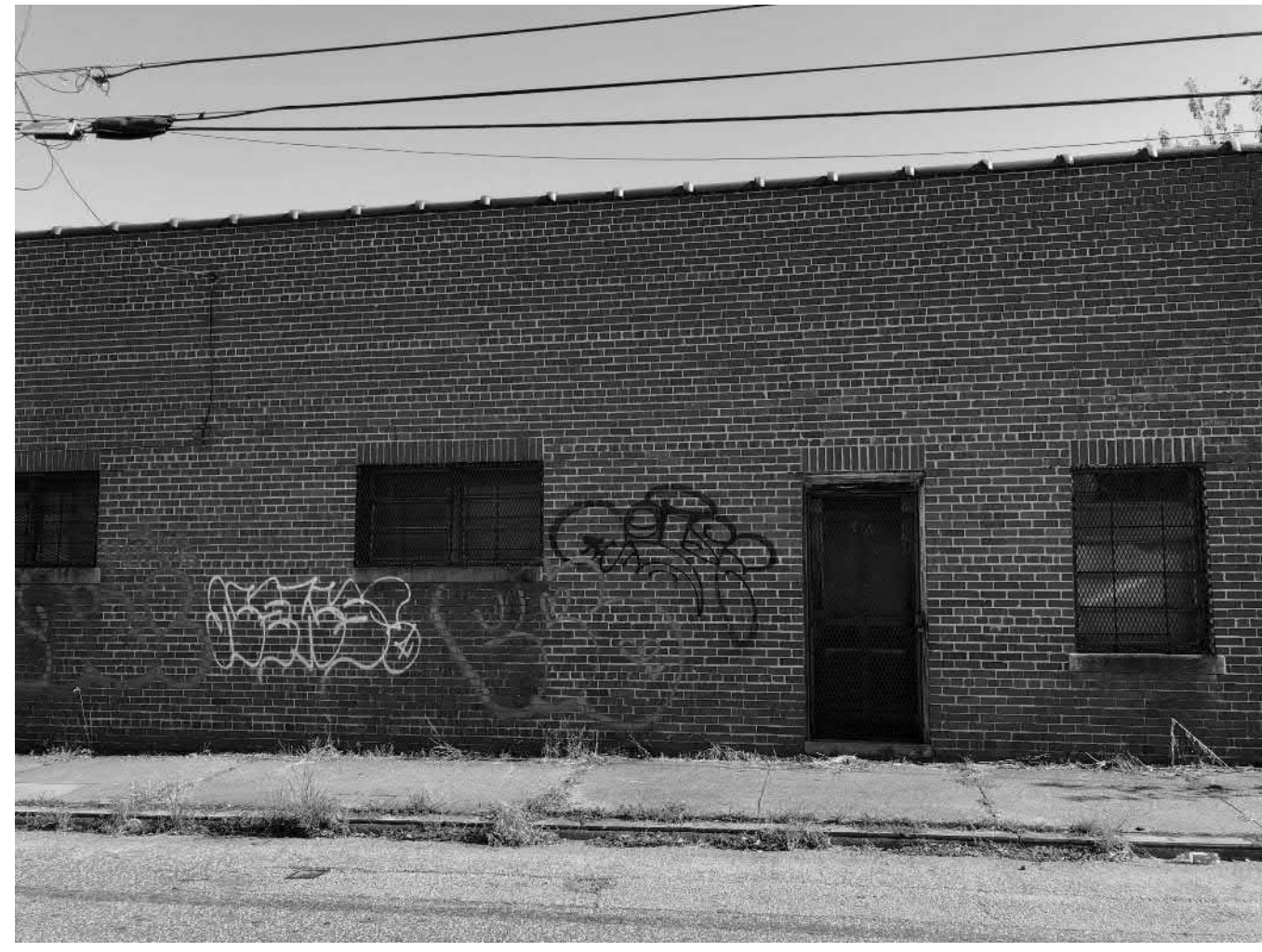
2. CLEAN EXISTING GRAFFITI PER NPS GUIDELINES
