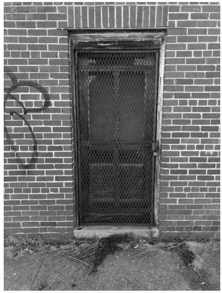
14. REPAIR, RESTORE & REFINISH DOORS SCHED. FOR REUSE.
