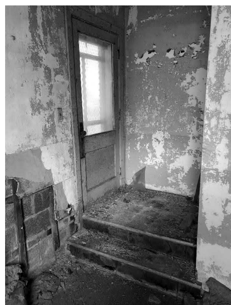
24. REPAIR INTERIOR FINISHES & PREP TO RECEIVE NEW CONSTRUCTION.
