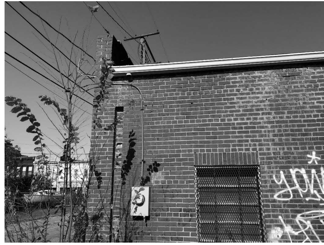
1. CLEAN, REPAIR, & REPOINT EXTERIOR MASONRY
