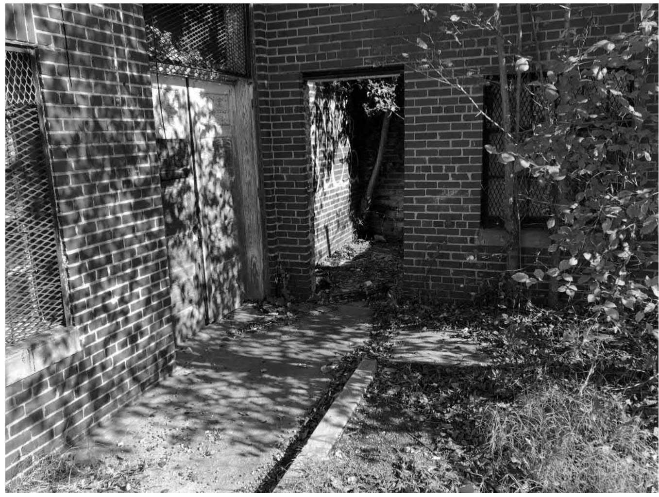
12. REPAIR, RESTORE & REFINISH DOORS SCHED. FOR REUSE.
