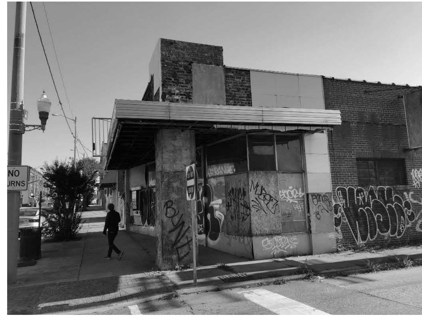
3. REMOVE EXISTING TILE CLADDING, CLEAN & REPAIR UNCOVERED MASONRY & PREP TO RECEIVE NEW MATERIAL. PROVIDE NEW TILES TO MATCH EXISTING OR PROVIDE ALL NEW TILES OF SIMILAR STYLE IF REPLICATED TILES ARE NOT AVAILABLE.
