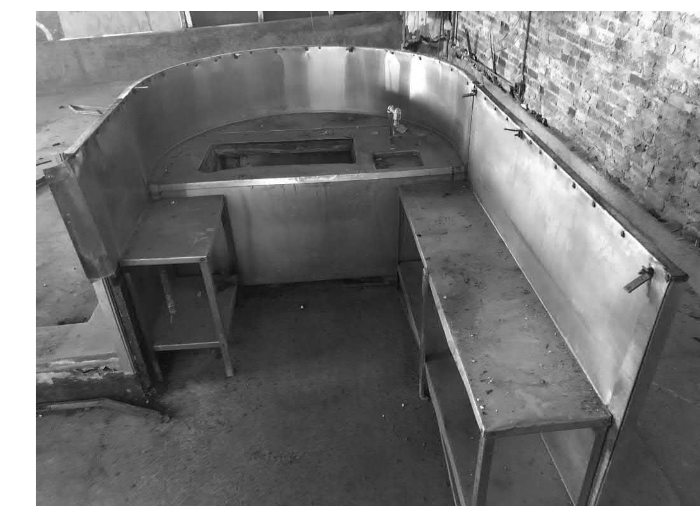
23. REPAIR DAMAGED COMPONENTS OF BOOTHS & COUNTERS. PROVIDE NEW, SIMILAR COMPONENTS WHERE REQ'D.
