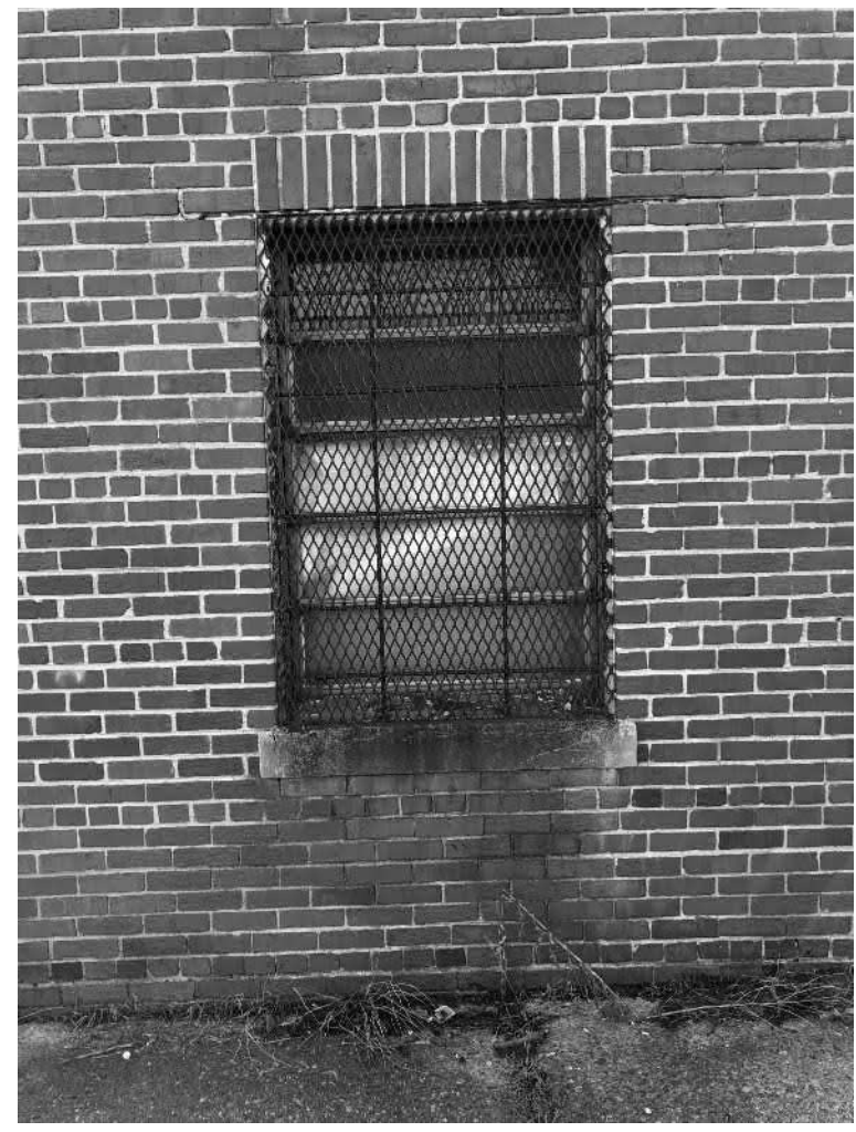
13. CLEAN & REPAIR MASONRY HEADERS & STONE SILLS.
