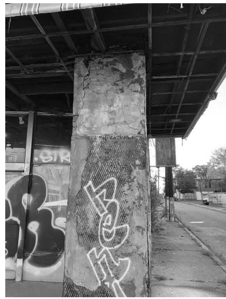
10. REPAIR, REPOINT, & RESHORE MASONRY COLUMN.
