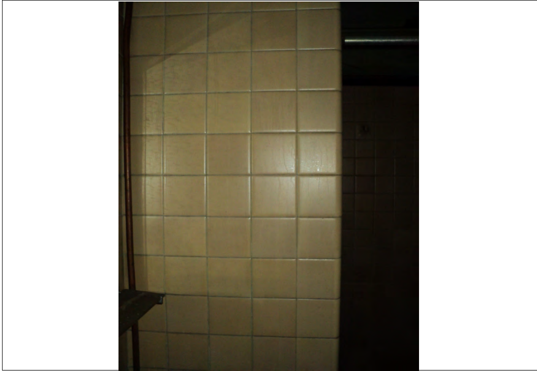
Photograph No. 17 Tan Ceramic Glazed Wall Tile (XRF Shot # 97)
