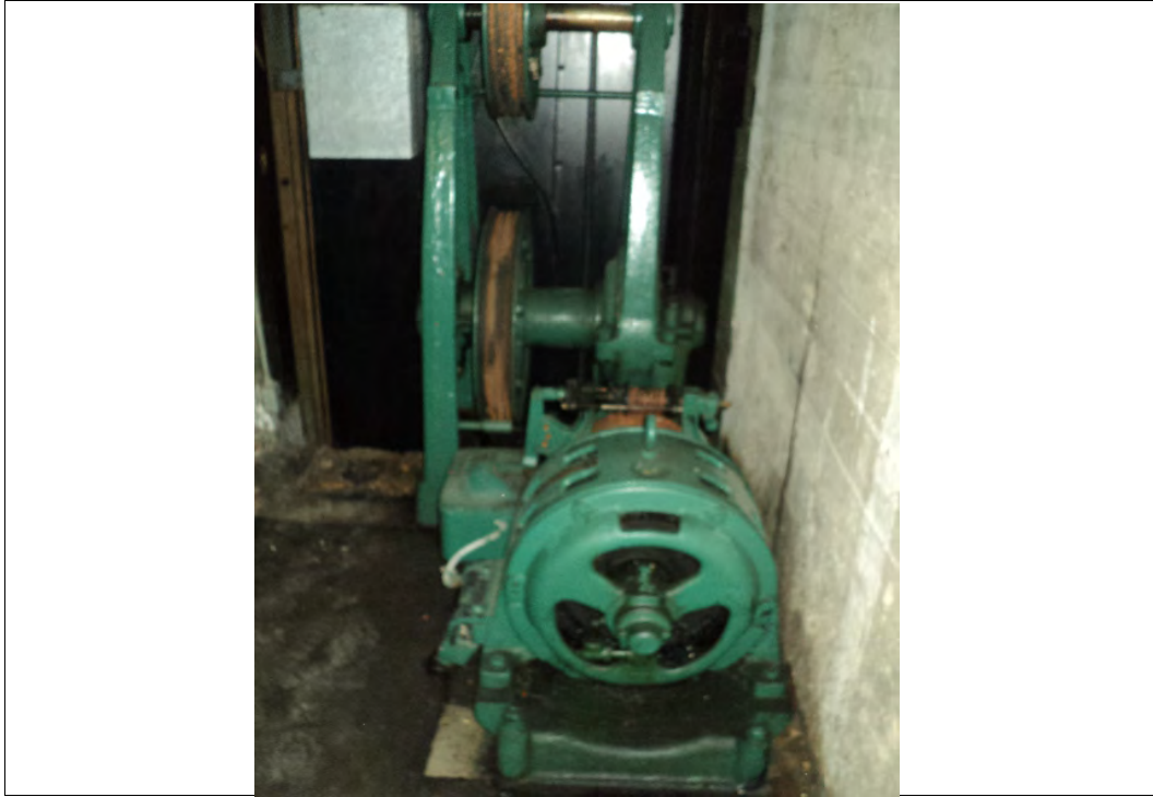
Photograph No. 11 Green Painted Metal Elevator Motor Equipment (XRF Shot #'s 73 & 74)
