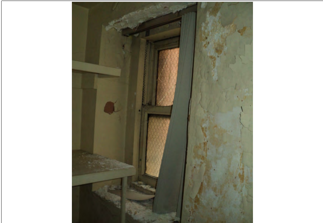
Photograph No. 18 Cream Painted Metal Window Components (XRF Shot #'s 158-159)
