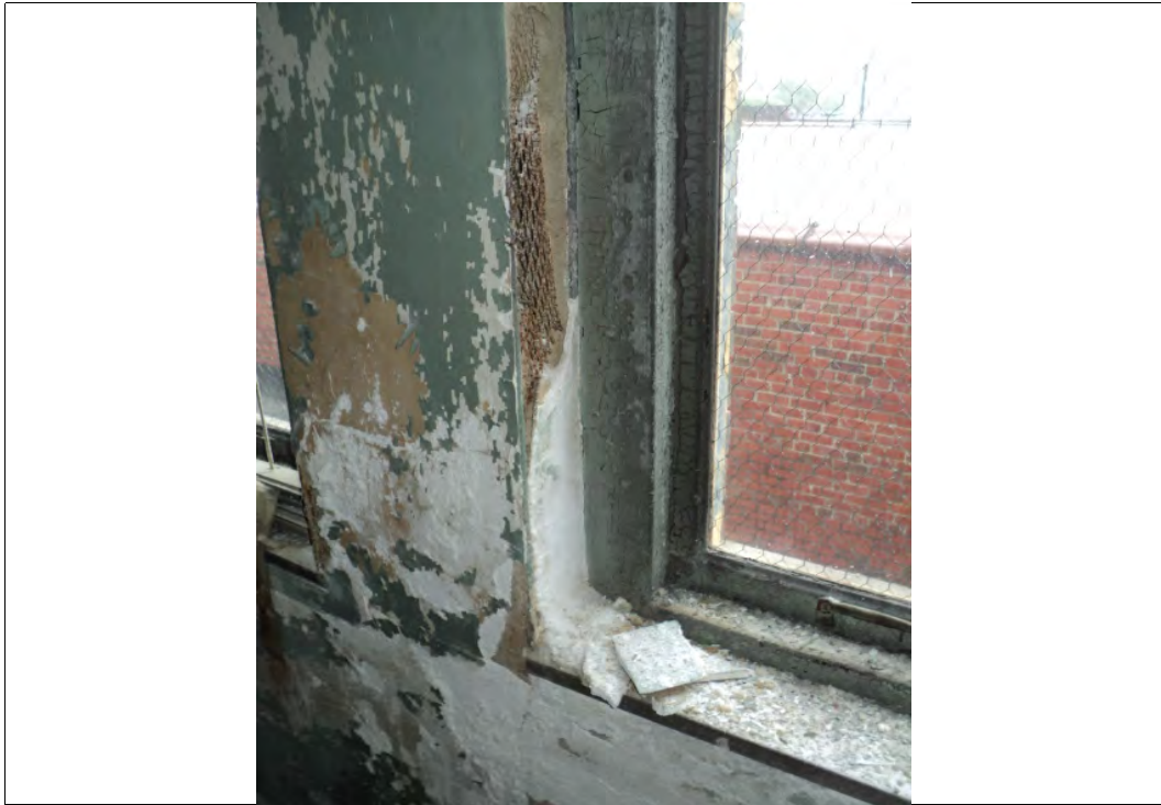
Photograph No. 32 Gray Painted Metal Window Components (XRF Shot #'s 250-251)
