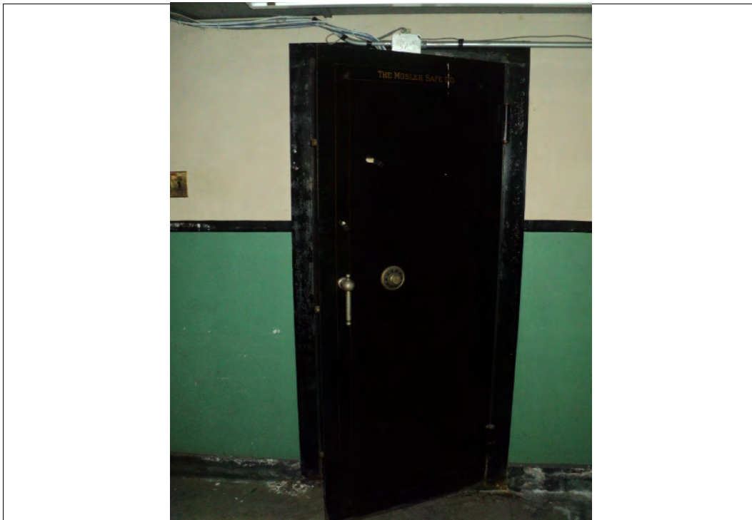
Photograph No. 7 Black Painted Metal Vault Door & Casing (XRF Shot #'s 47 & 48)
