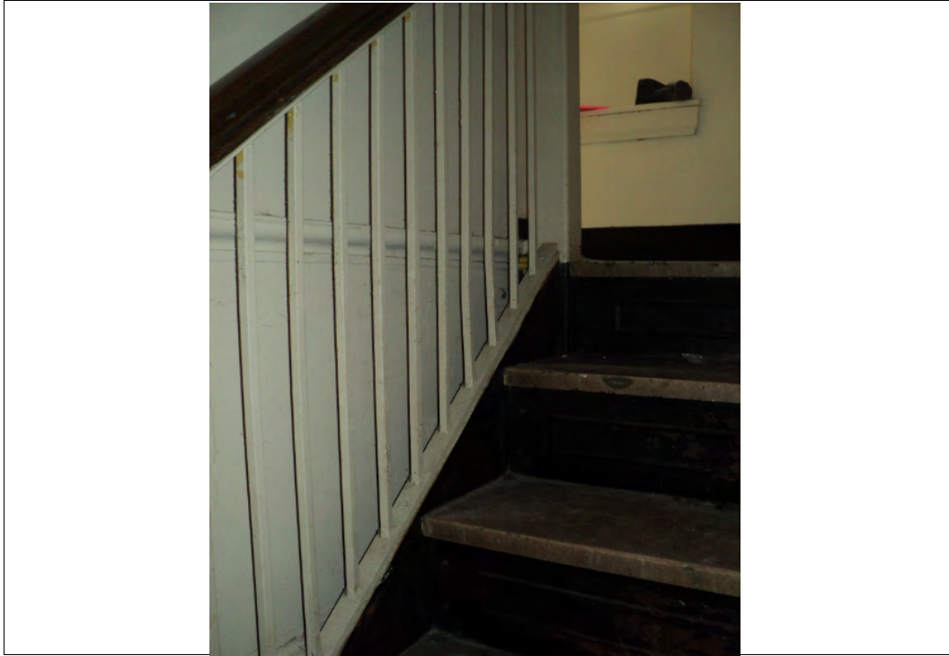
Photograph No. 19 Cream Painted Metal Stair Components (XRF shot #'s 165-166)
