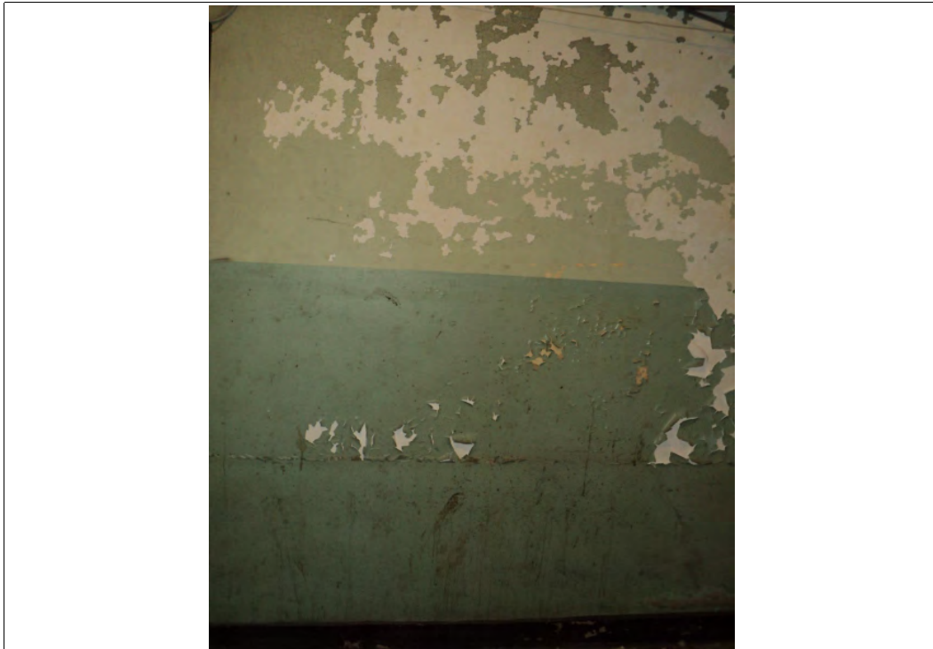
Photograph No. 10 Dark Green Painted Plaster Walls (XRF Shot #'s 69,80,91,170 & 253)
