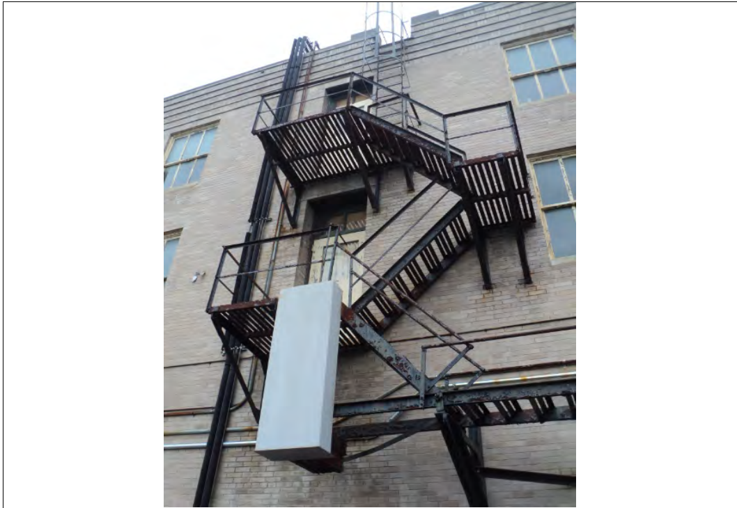
Photograph No. 1 Black Painted Metal Fire Escpae Components (XRF Shot #'s 4-8)
