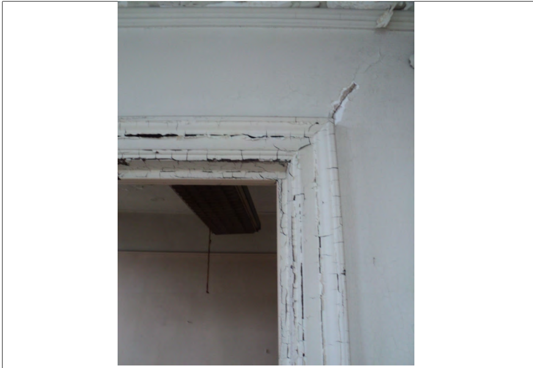
Photograph No. 34 Gray Painted Metal Door Casing (XRF Shot # 277)
