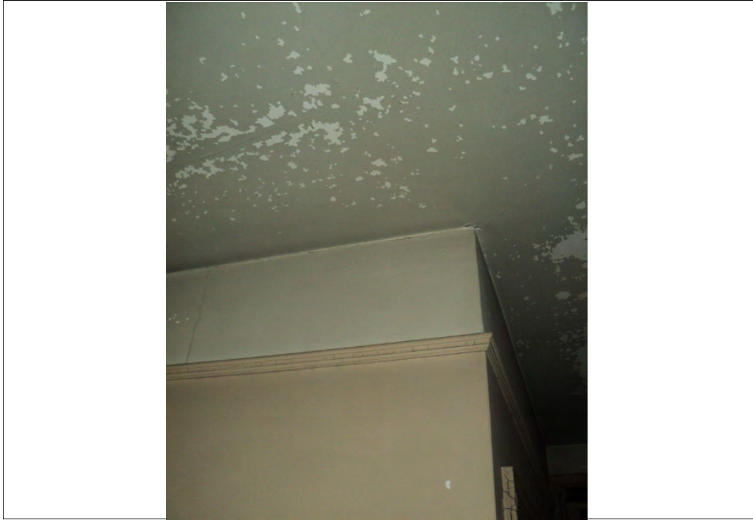
Photograph No. 33 Cream Painted Plaster Wall (XRF shot # 265)
