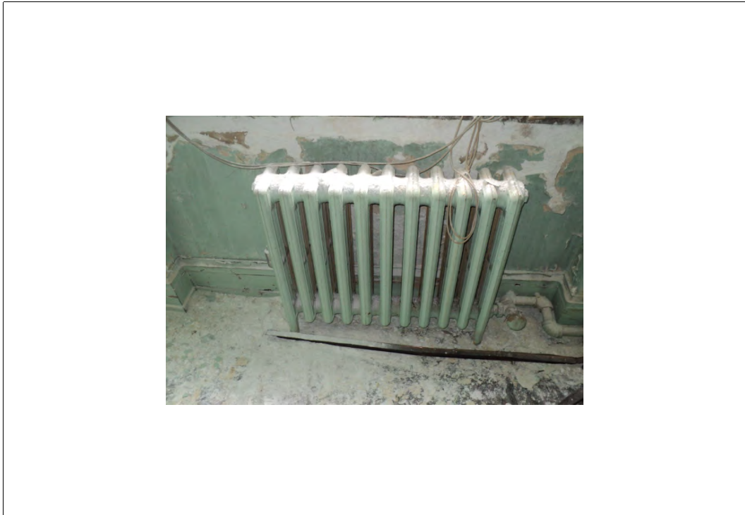
Photograph No. 22 Green Painted Metal Radiators (XRF Shot # 184)
