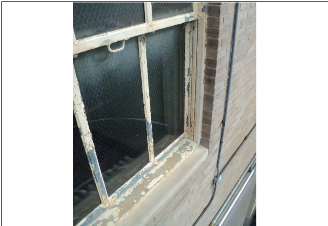
Photograph No. 2 Cream Painted Metal Exterio Window Components (XRF Shot #'s 9-12)
