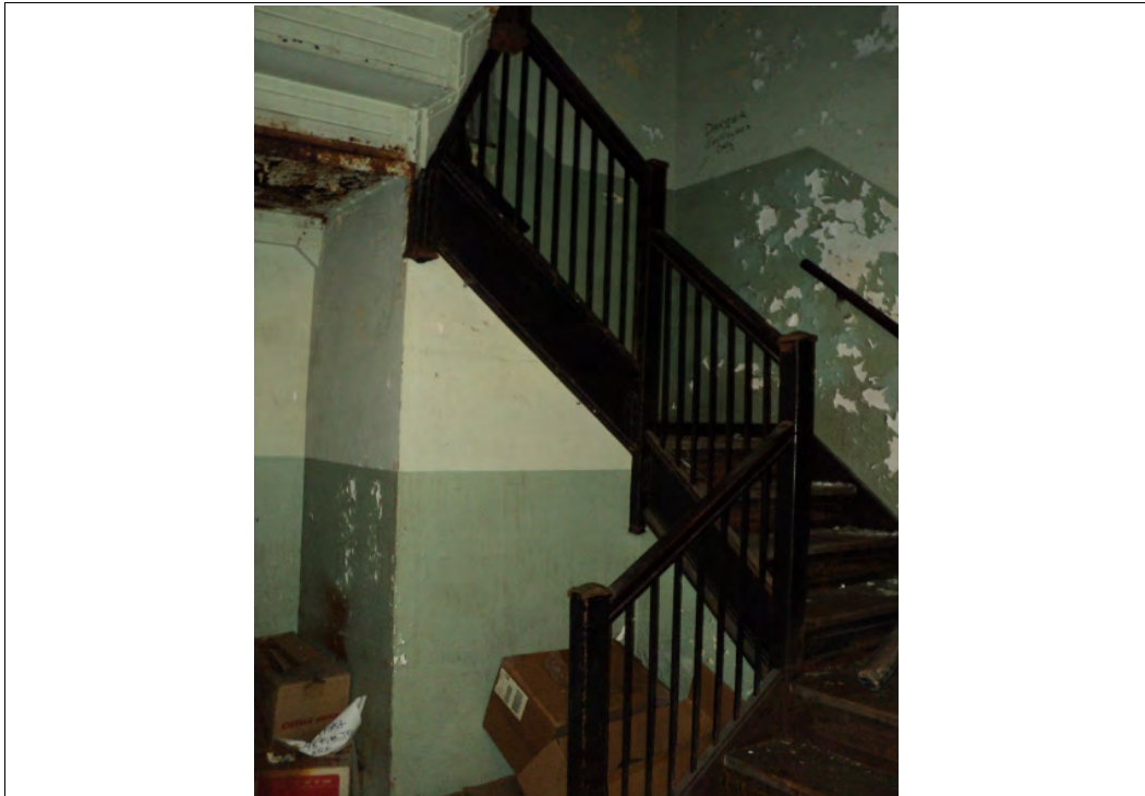
Photograph No. 13 Black Painted Metal Stair Components (XRF Shot #'s 81,83,85,167 & 168)
