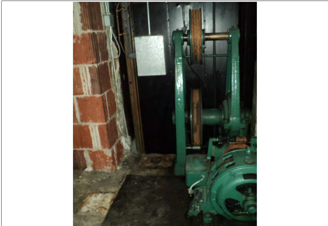
Photograph No. 12 Black Painted Elevator Car Exterior Walls (XRF Shot # 75)
