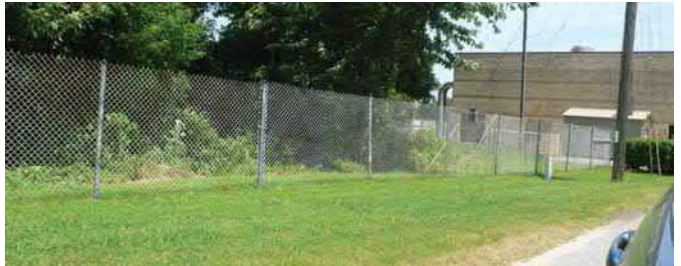
Fence at Wastewater Treatment facility
