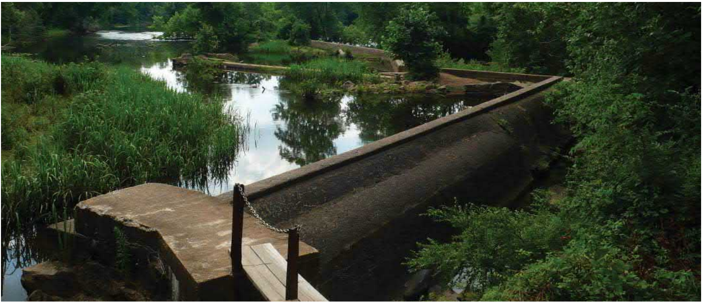
Historic Abutment Dam
