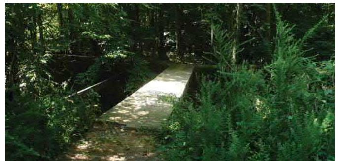
Existing footbridge across canal
