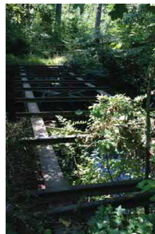
Existing bridge frame
