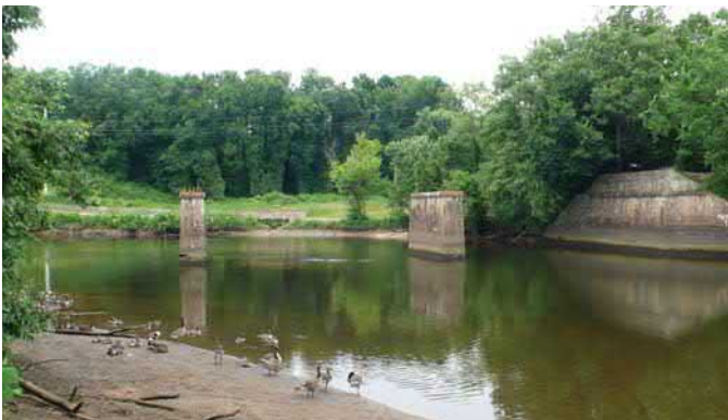
Existing bridge abutments
