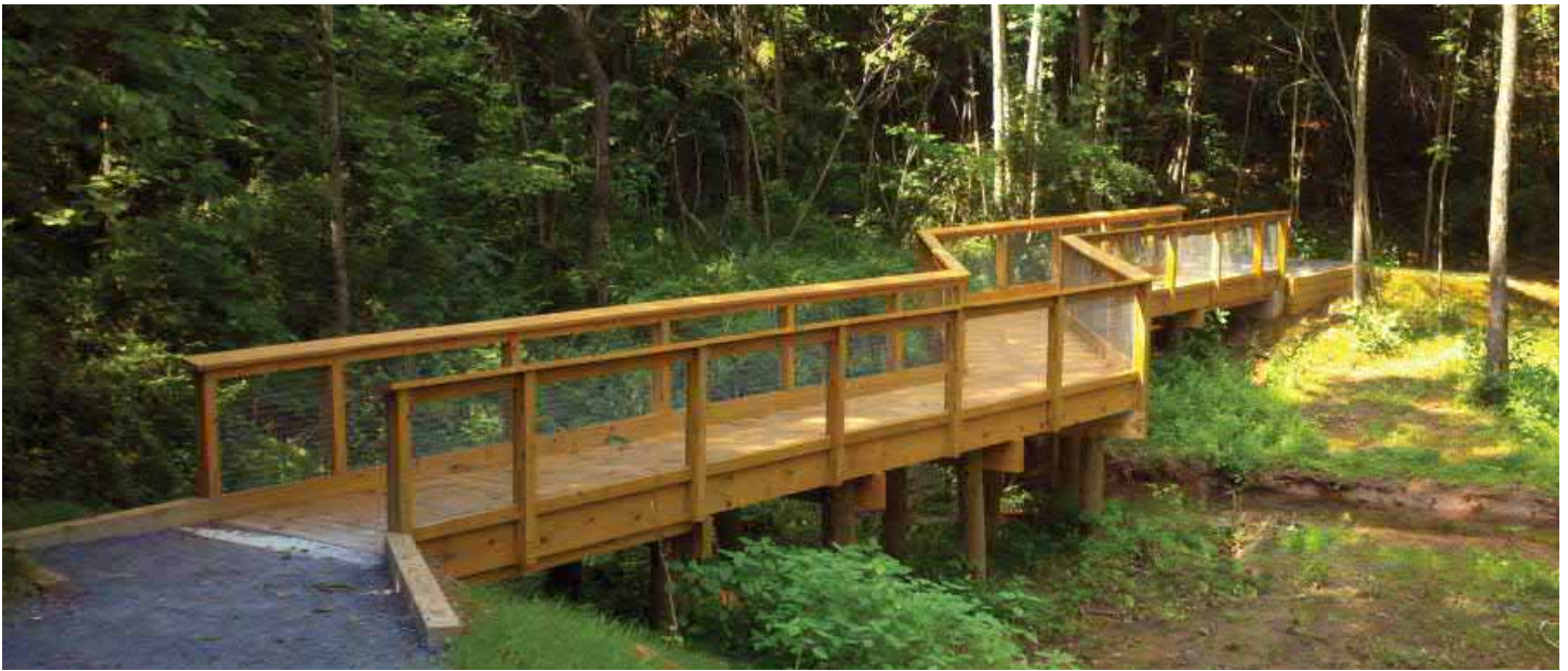
Example of rustic trail bridge
