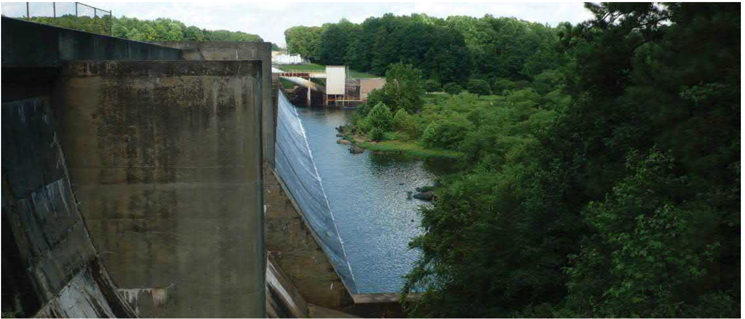
Dam at Lake Chesdin
