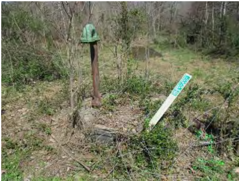
Site Photograph 8 – Sewer vent and cleanout on the western portion of the Property
