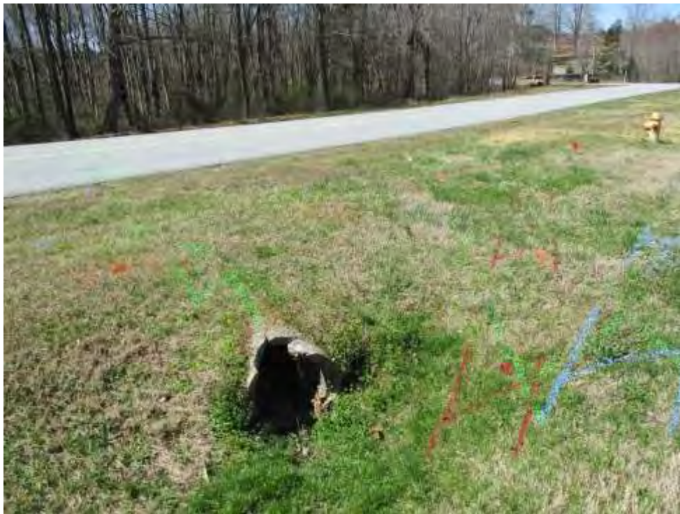
Site Photograph 6 – Culvert on the southern portion of the Property
