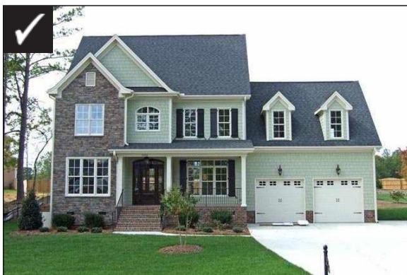
Recessed garage with individual doors
