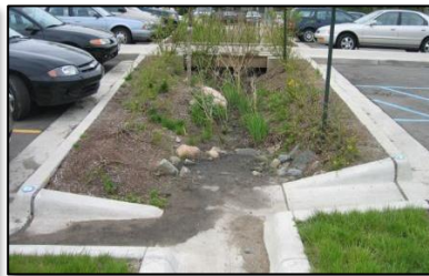
Curb and gutter with curb cuts directed to landscaped area
