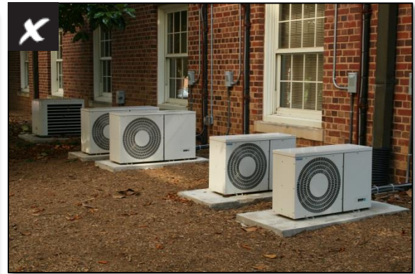
Unshielded ground-level equipment
