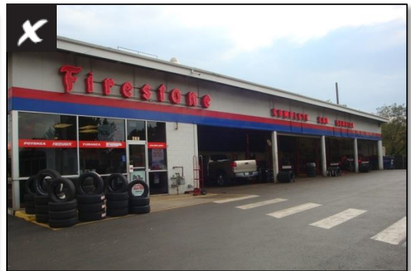
Service bays on primary building wall
