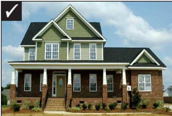
Elevated brick foundation
