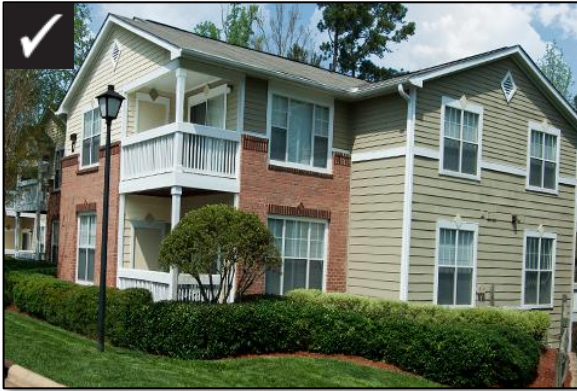
Adequate windows with regular rhythm and alignment
