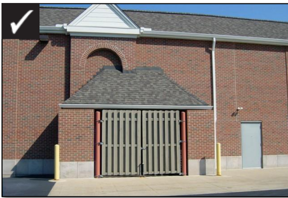
Screened ground-level equipment
