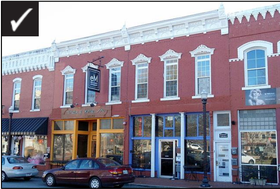
Brick façade with bright accents
