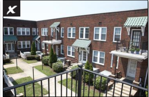
Flat roof with no decorative parapet or variation
