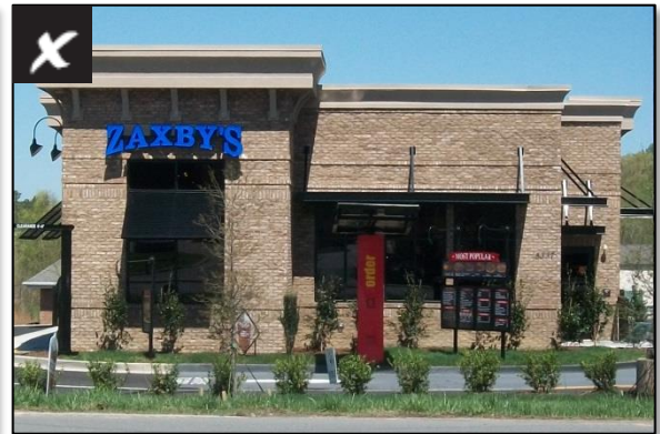
Drive-through ordering station on front facade
