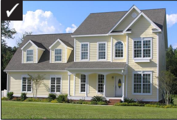
Adequate windows with regular rhythm and alignment
