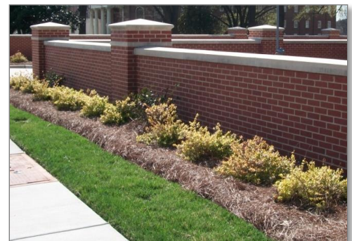
CBD Parking Lot Screen Wall
