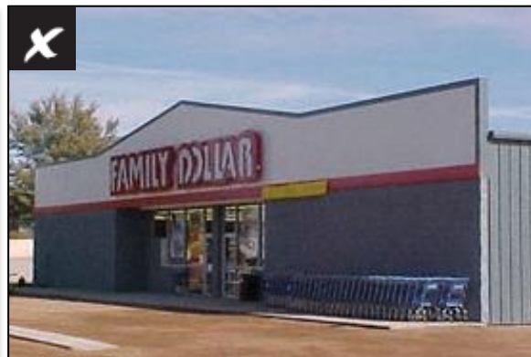
Painted concrete block and metal facades
