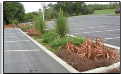
Recessed curb with sheet flow drainage to landscaped area
