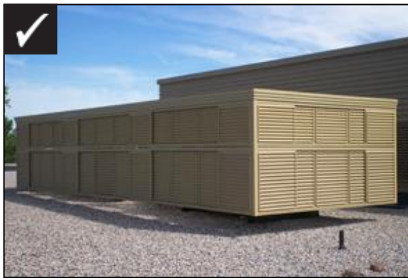
Screened roof-top equipment
