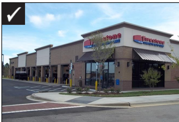
Service bays on secondary building wall
