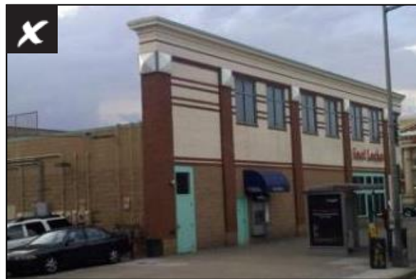
Non-continuous false front parapet without height changes
