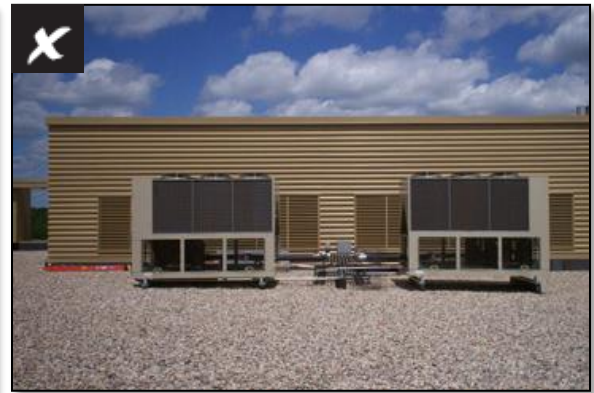
Unshielded roof-top equipment
