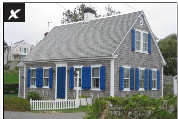
Large expanse of roof without variation
