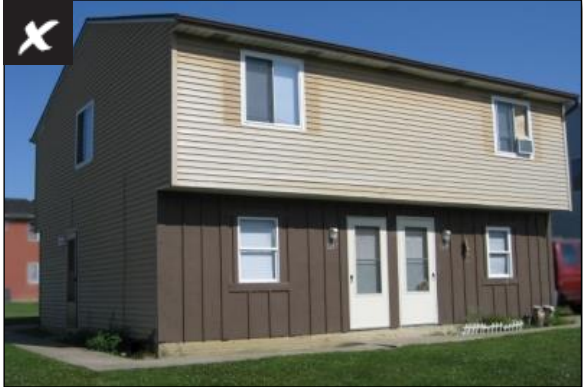
Entrances on same plane of facade
