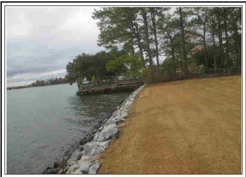
VIEW OF THE LAFAYETTE RIVER / RIP-RAP BULKHEADING
