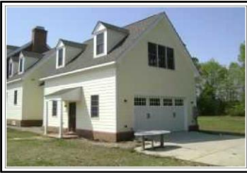
Right Side of Subject House
