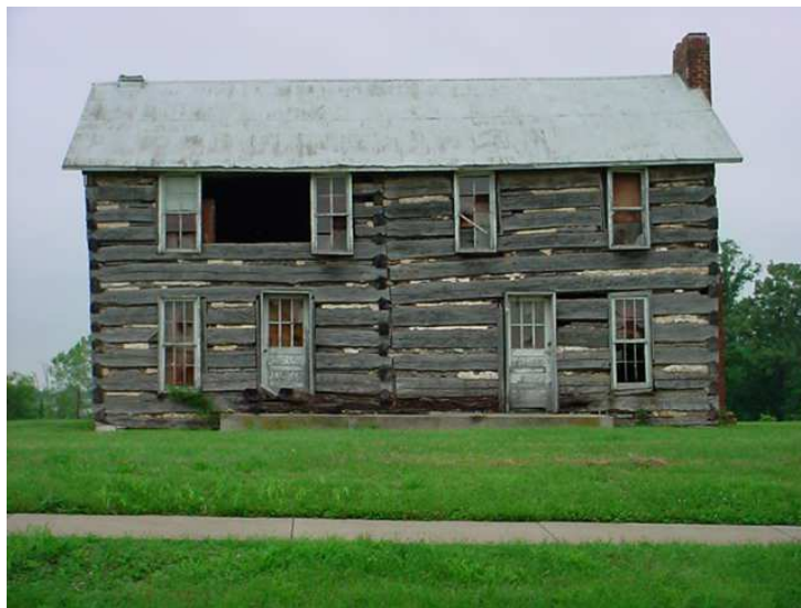
The Edwin Stovall House survived tornado damage in 1914.
