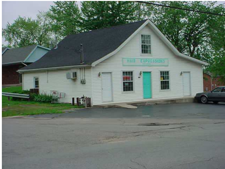
The Stoney's Grocery building is the only example of old-style country general stores that still remains in Radcliff.
