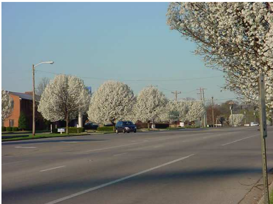
Lincoln Trail Boulevard is classified as a minor arterial, due to the fact that it is not a limited access roadway.
