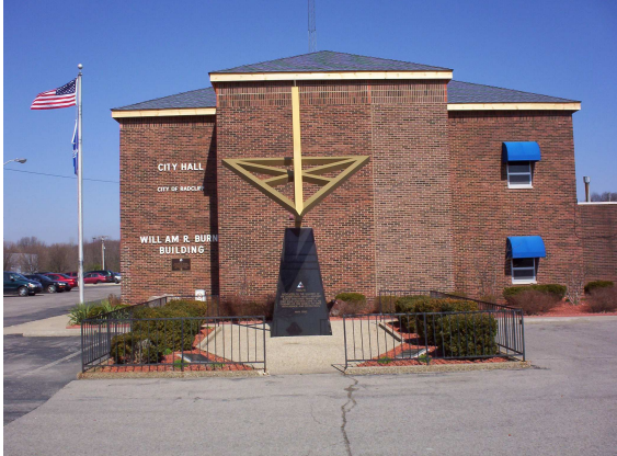
Pictured above is Radcliff City Hall. A new roof is currently being put on the building.
