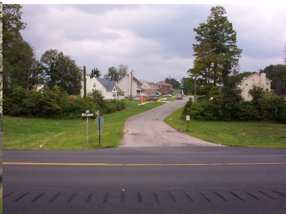
Skyline Drive is classified as a collector road, because it collects traffic from local roads in the Hilltop Terrace Subdivision and it channels this traffic onto arterial roads such as Joe Prather Highway, pictured above.
