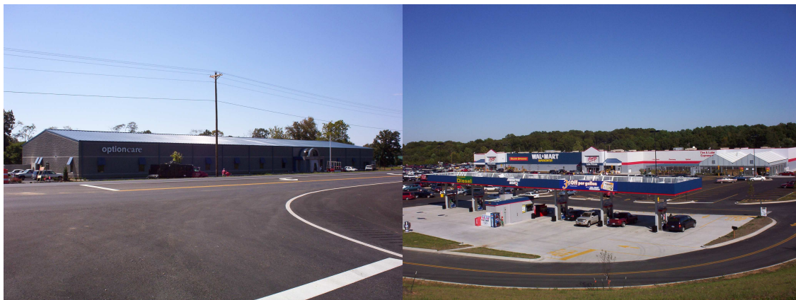
Pictured above, the Option Care Building is an example of the growing manufacturing industry in Radcliff. This recently constructed 184,000 square foot Wal-Mart Supercenter is a sign of strong retail trade in Radcliff.
