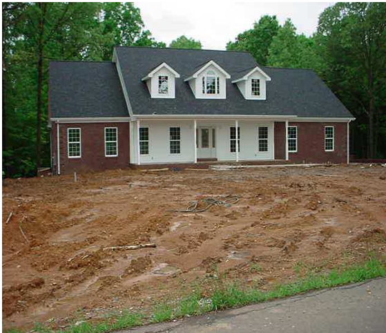
This home is being constructed in an RU-E Zone, which experienced significant growth due to annexation.
