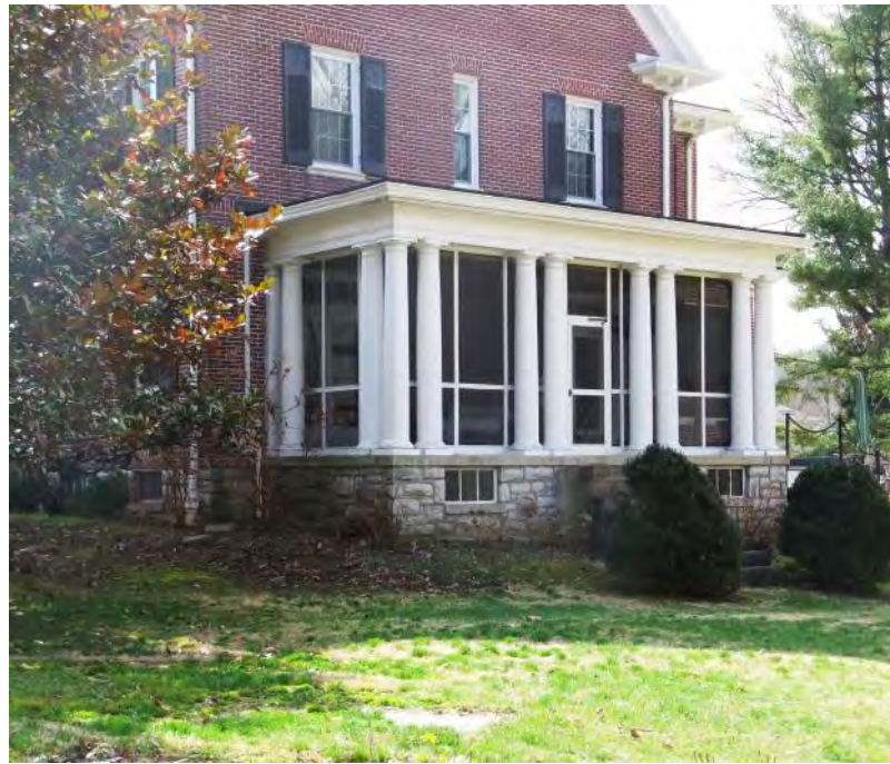
When enclosing historic porches on secondary elevations, it is important to leave original columns and trimwork in place. Also, using full-height glass or screen panels helps preserve the sense of transparency and openness associated with a porch so that it does not appear as a closed-off room.
