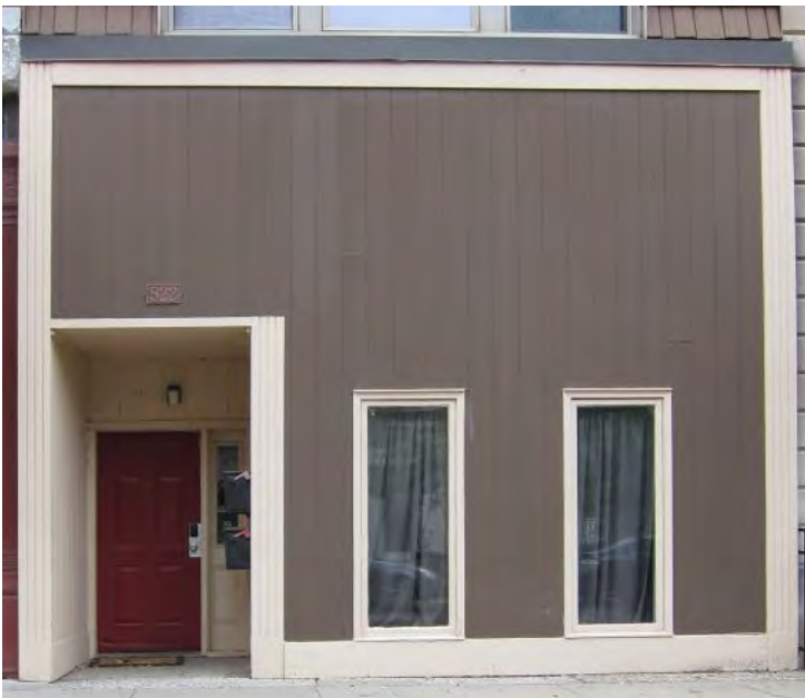
Storefronts are critical components of the pedestrian streetscape. Unsympathetic alterations can severely impact the character of a space and limit opportunities for interactions with patrons.
