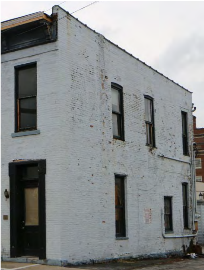
Locating service connections at the rear of secondary elevations as illustrated above is the most appropriate means of locating utilities within the historic district.
