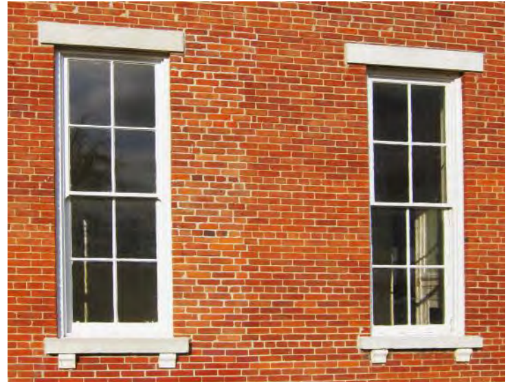
Repointing that does not match the characteristics of the original mortar can cause it to stand out from the surrounding masonry, detracting from the aesthetic of the building, as is shown above where cement-rich, bright white mortar was used to repoint the mortar around the window to the left.
