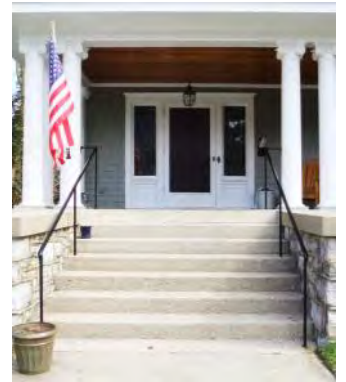
This residence appropriately uses a simple metal handrail with minimal supports, which minimizes the railing against the backdrop of the porch.
