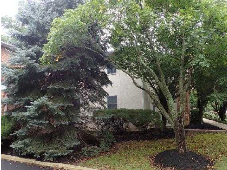
Rear elevation Exterior Surface
