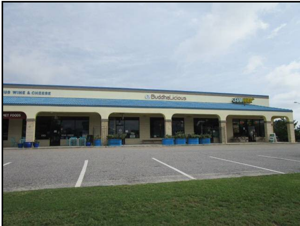
Subject View Facing Northeast
