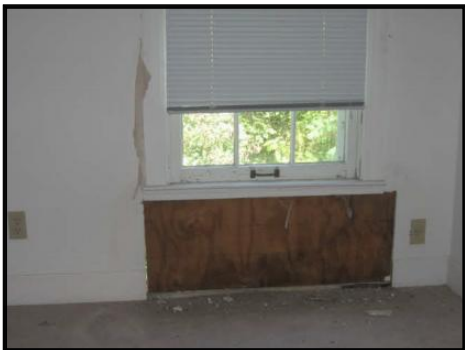
HVAC unit removed
