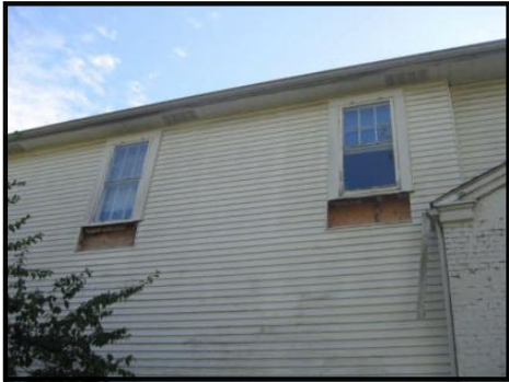
HVAC units removed
