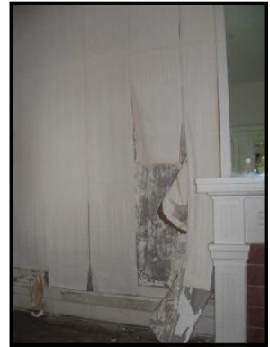
walls need repair
