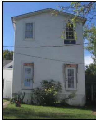
HVAC unit removed, doors installed
