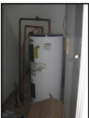
m. Bdrm water heater
