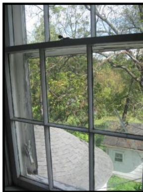
multiple windows trim needs repair
