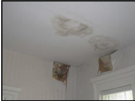
walls need repair
