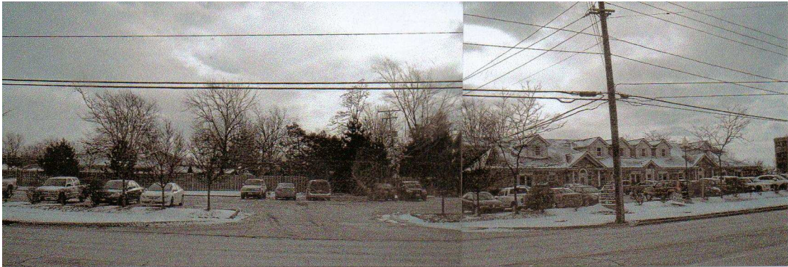
FRONT VIEW OF SUBJECT CONDOMINIUM AND PARKING LOT
