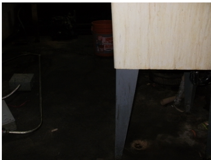
Stained floor and floor drain beneath sink
