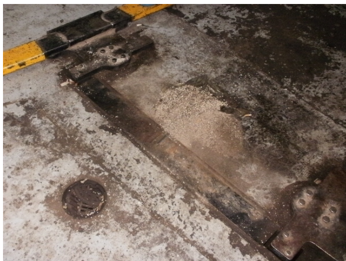
Staining in and around drain by hydraulic lift. It is unknown where the drain leads
