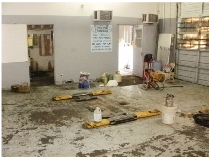
Southern hydraulic lift and drain, looking southwest. West door leads to office and east door leads to compressor room
