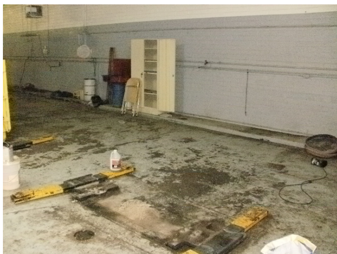
Southern portion of automotive repair area. Note hydraulic lifts, staining on ground, and drain
