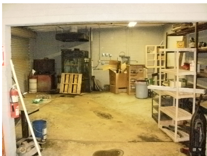
Storage area in western portion of addition. Note floor drainage into full sump by the pallet. Looking west.
