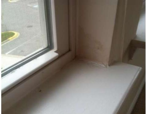
2403. Walls Repair/Replace/Monitor. Drywall. Cracking observed in drywall/plaster. Noted in master and family room.
