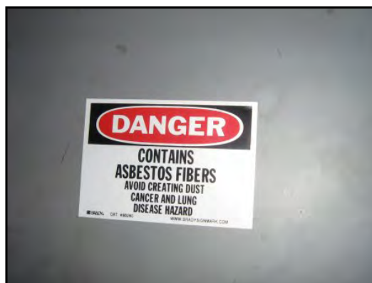
24 : ACM warning label on door to room at Project
