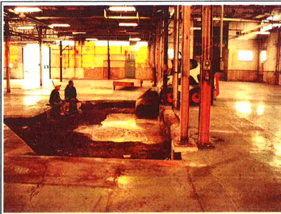
Photo No. 6: Pouring slurry into the excavation.
