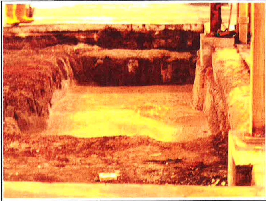
Photo No. 7: Slurry in the excavation.
