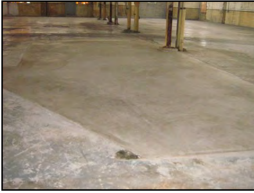
25 : Area of former PCB remediation capped with new concrete
