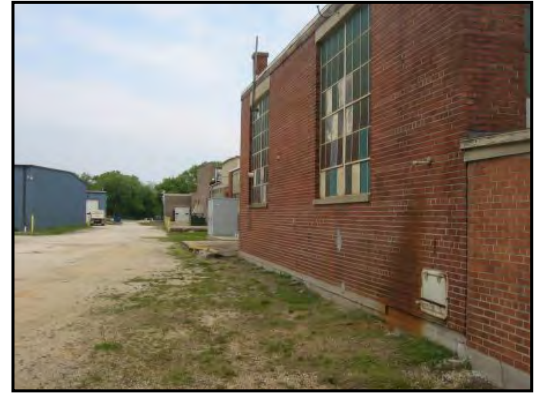
2 : Along the alley and south side of the manufacturing building
