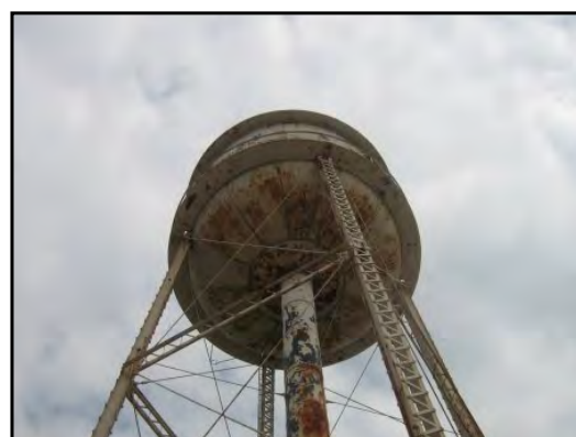
10 : Water tower located on the north side of the Project
