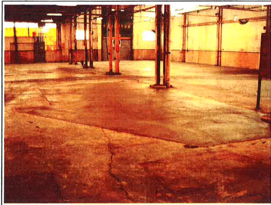
Photo No. 16: Finished concrete cap.
