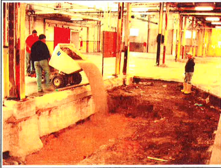
Photo No. 5: Pouring 1,200 lb/in 2 compressive strength slurry into the excavation.
