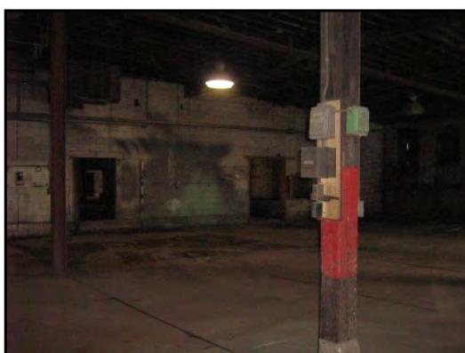
21 : Interior of foundry building
