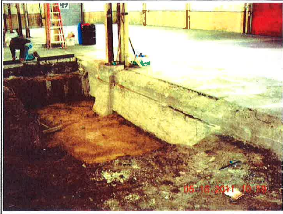
Photo No. 3: Installing No. 4 steel dowels in the concrete slab.
