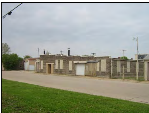
5 : East side (along Locust) of original portion of Project building
