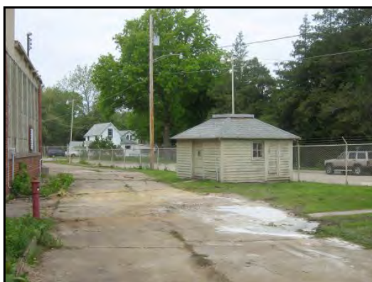
11 : Pump house located on the north side of the Project
