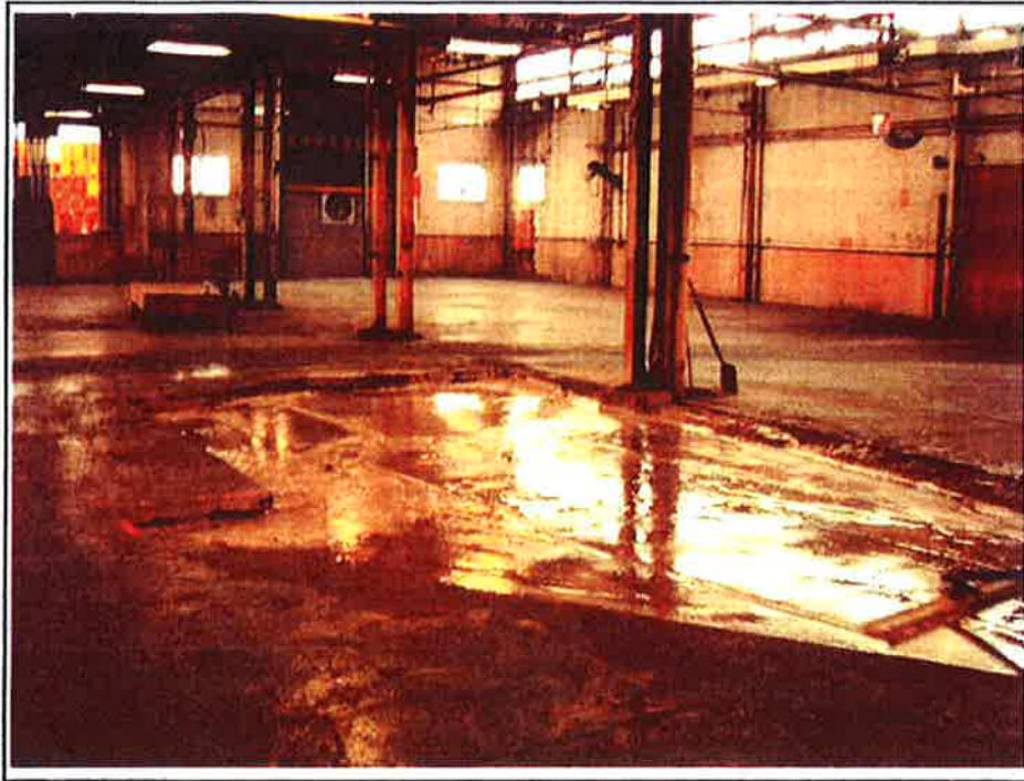
Photo No. 9: Floating flowable slurry in the excavation.
