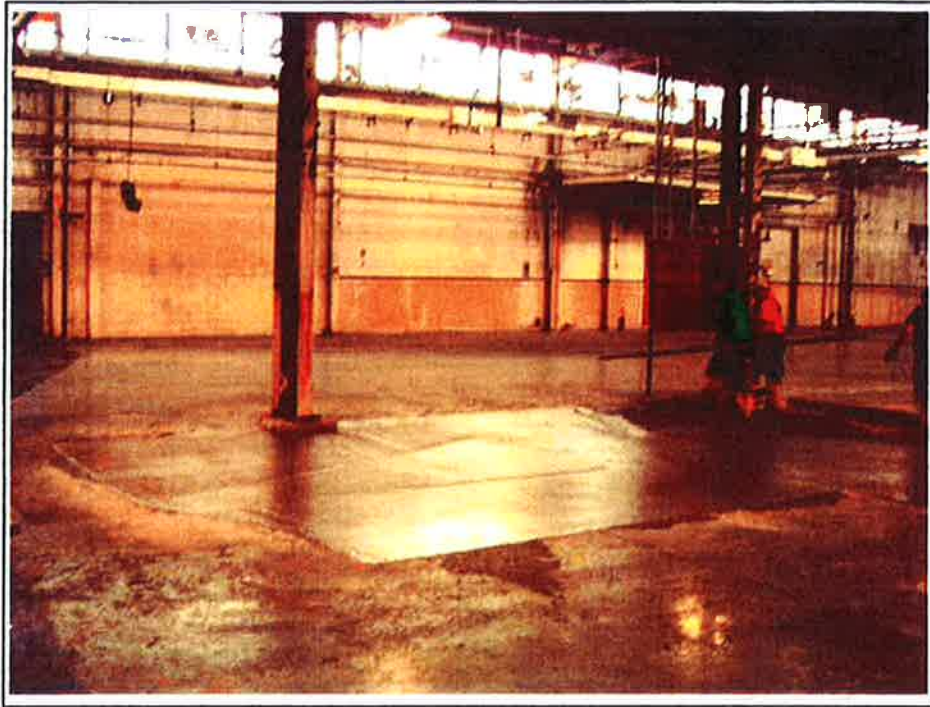
Photo No. 13: Concrete cap installation.
