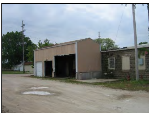
9 : Storage building north of the foundry building
