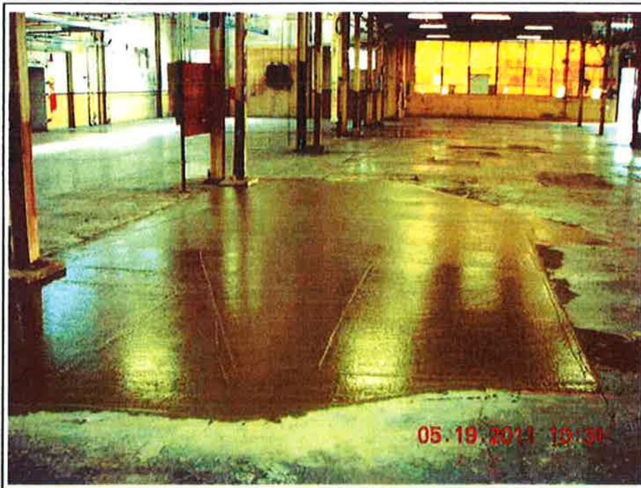
Photo No. 14: Installed 6-inch concrete cap.
