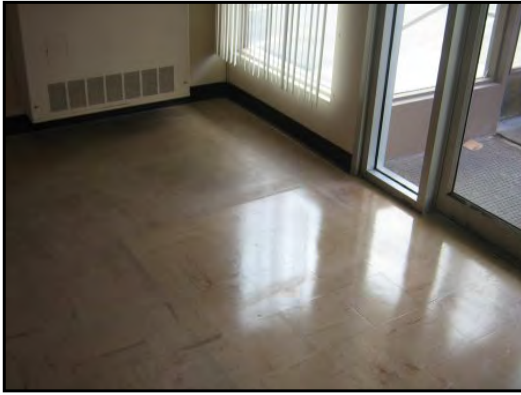
13 : Floor tiles in office area
