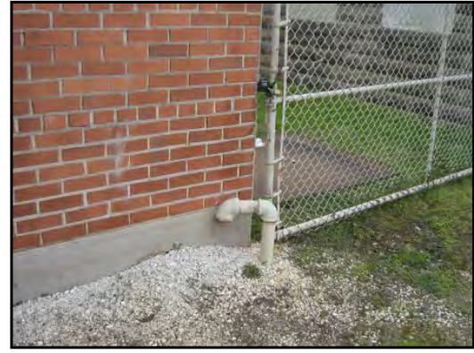
26 : Unknown pipe located on south exterior of manufacturing building
