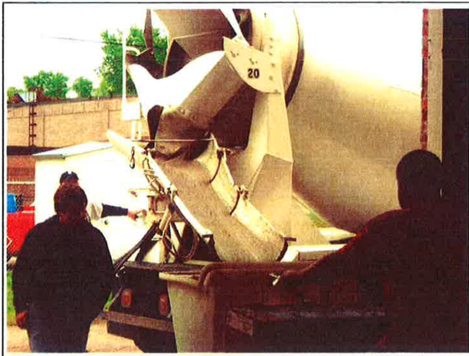
Photo No. 4: Flowable slurry decanted to mobile tote.
