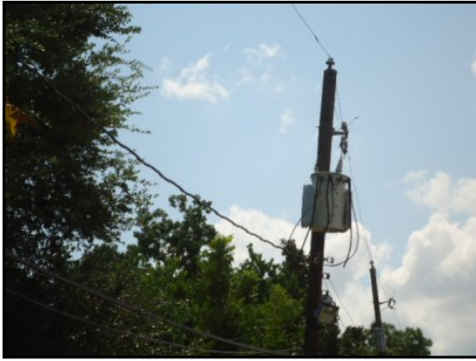
19 : Pole-mounted transformer
