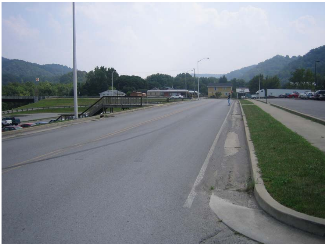
VIEW OF THE SYKES BLVD. ELEVATION & FRONTAGE
