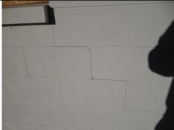
CRACKS IN EAST WALL
