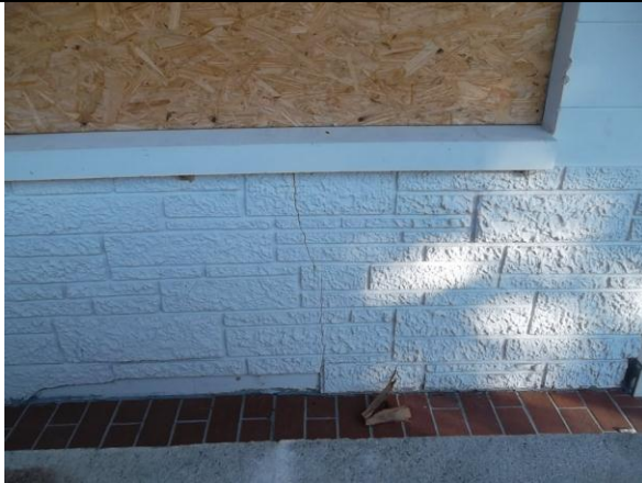
CRACKS IN SOUTH WALL
